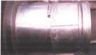
Coupling Hub before Repair
