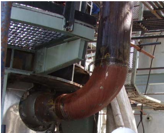
New Synthesis Gas Converter (108-D) Elbow (14" NB x Sch120, P22 material Elbow)
