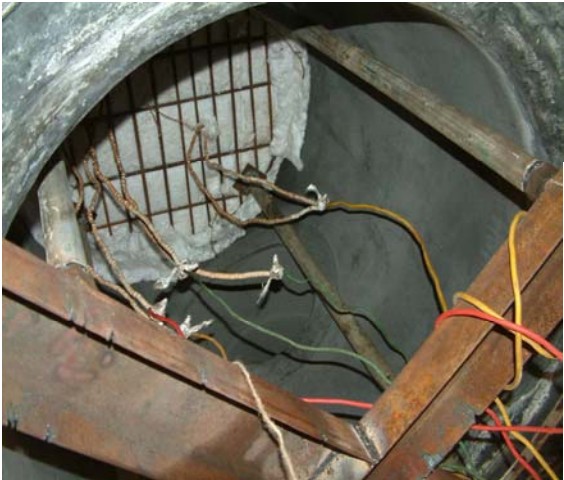
Photograph for arrangement of heating coil in bottom channel cover
