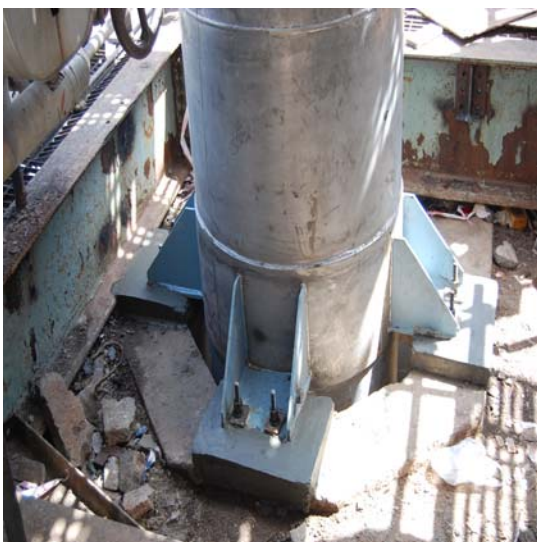
FIG 12 , Foundation of new shell
