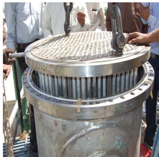
FIG 13 Tube bundle being inserted in new Shell
