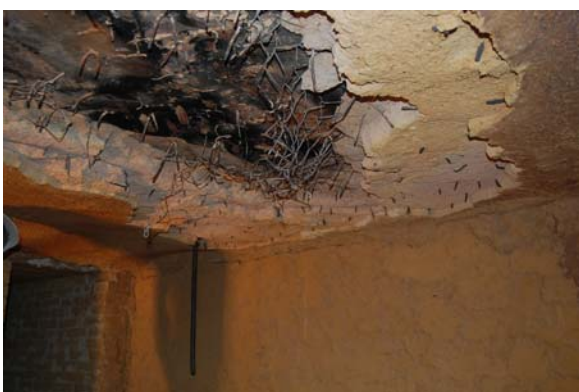
Damaged Roof Insulation of HT Convection zone
