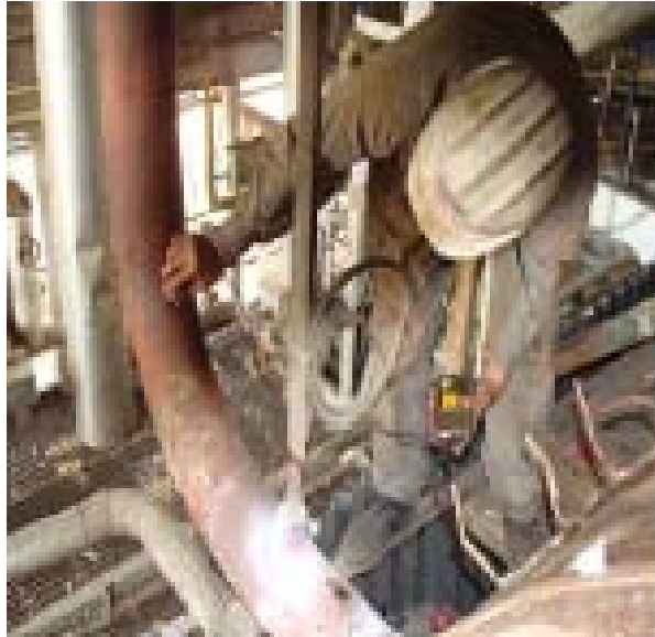
DPT of Feed water line attachment welds
