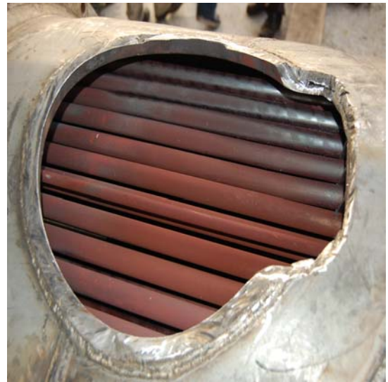
FIG 11 , Bulged portion of old shell near 14" Gas Inlet nozzle was cut and removed to facilitate tube bundle removal
