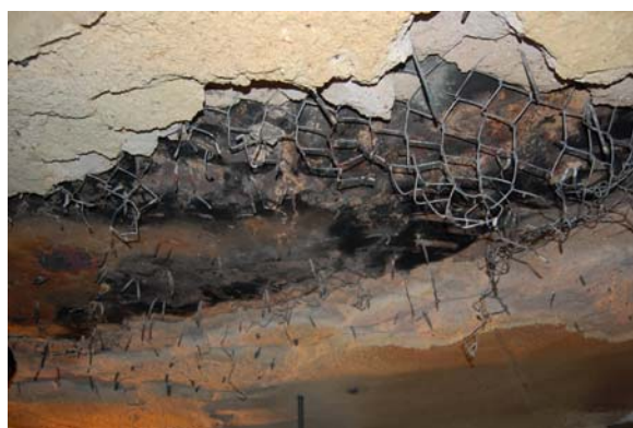
Damaged Roof Insulation of HT Convection zone
