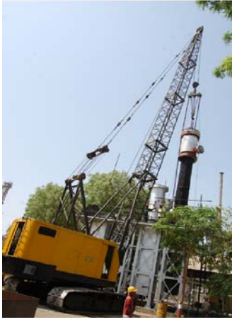
Spare Tube bundle being lifted for 101- CB
