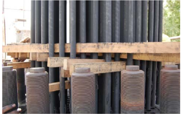
Inner tube being inserted into outer bundle for 101-CA
