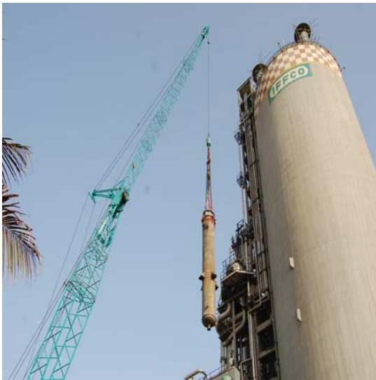
FIG 10 , Tube bundle with old shell lifted by Kobelco Crane
