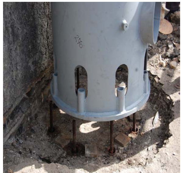
Figure – 31 : New bottom shell being kept on foundation
