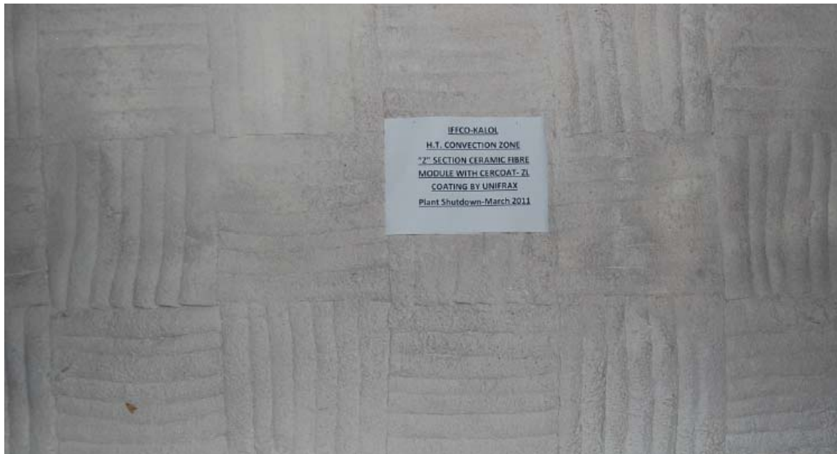
AFTER: NEW CERAMIC 'Z' SECTION INSULATION & CERCOAT ZL COATING
