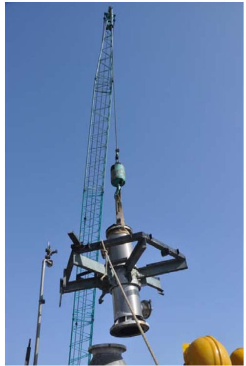
Figure – 28 : Top shell lifted by Kobelco Crane
