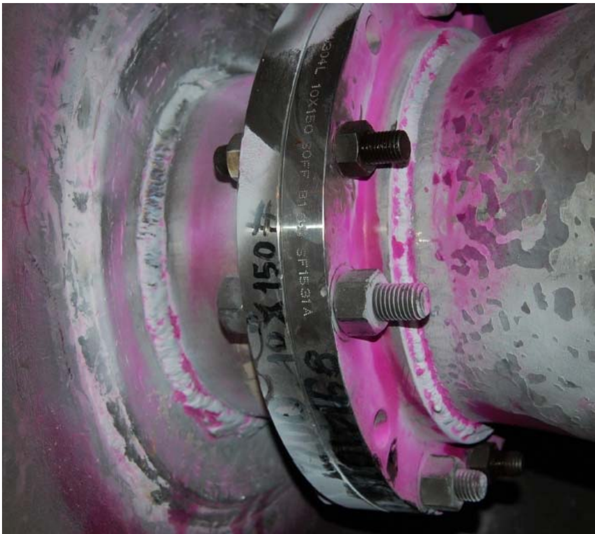
NEW 10" X 150# FLANGES ON THE INLET NOZZLE INSIDE THE VESSEL
