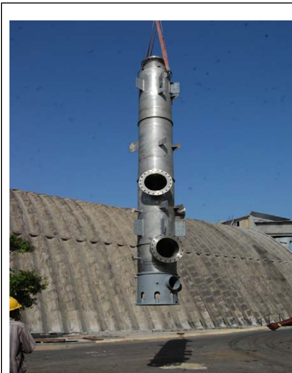
Figure – 30 : New bottom shell lifted by Kobelco Crane
