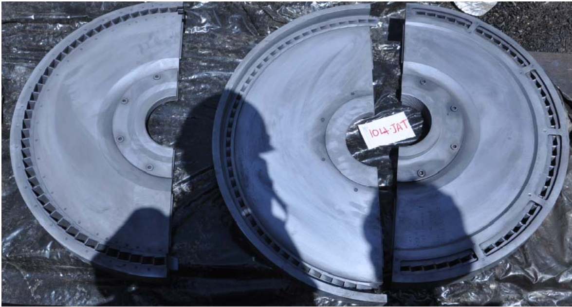
104-JAT DIAPHRAGMS CLEANING & INSPECTION UNDER PROGRESS
