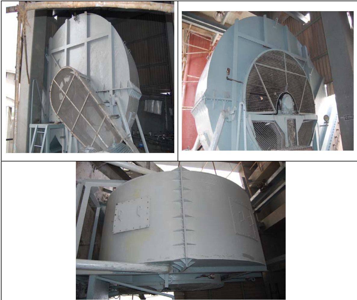
Figure – 32 : K-1701, After application of Chemical resistant coating
