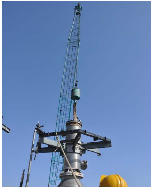
Figure - 27 : Kobelco Crane positioned for lifting top shell
