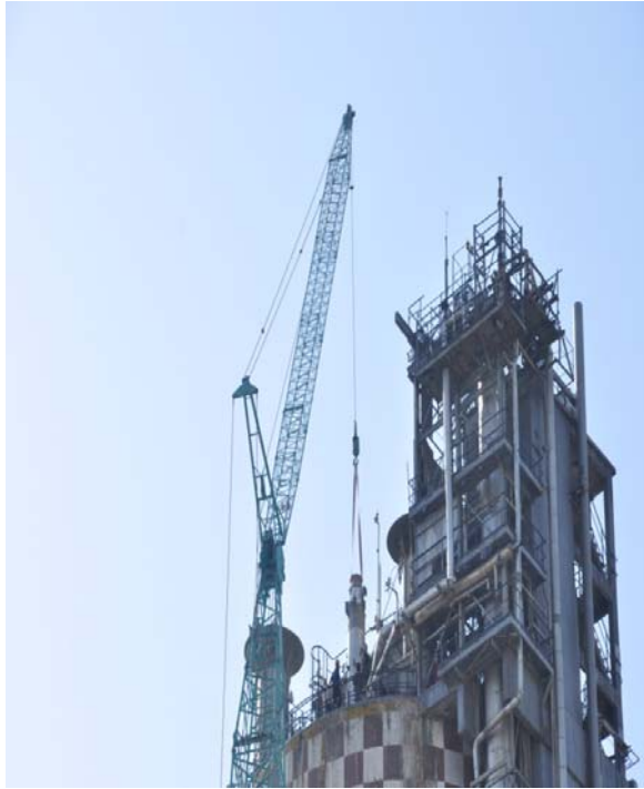
Figure – 29 : Kobelco Crane positioned for lifting bottom shell
