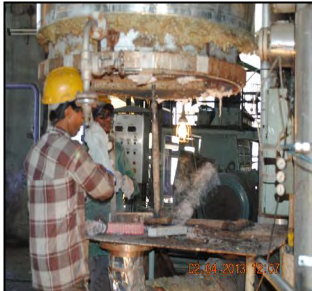
Removal of orifice plugs from bottom tube sheet
