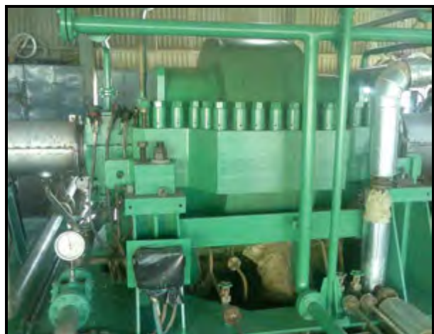
After overhauling of LP case
