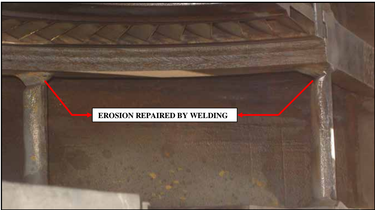
101-JT BOTTOM CASING DIAPHRAGM HOLDER REINFORCEMENT
