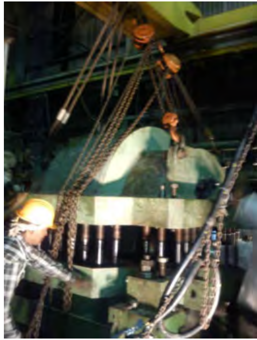
Lifting of top casing of LP case
