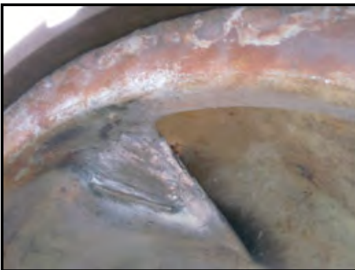
Repaired wane by welding
