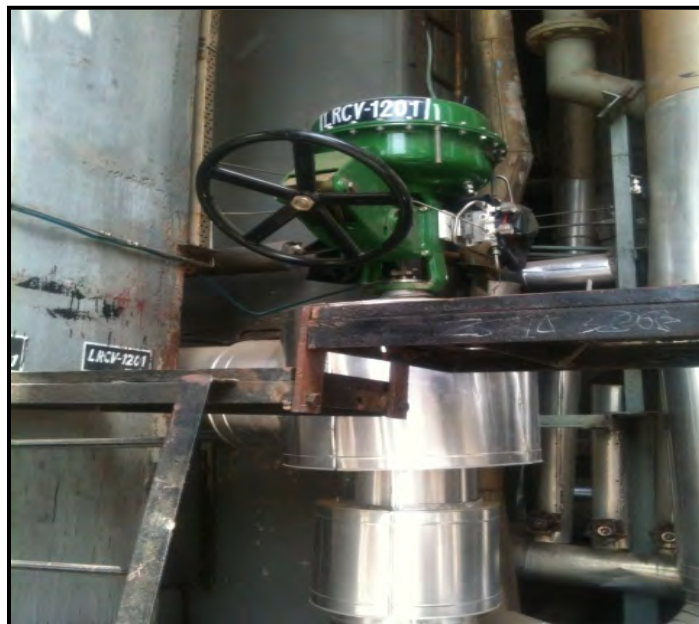
Newly installed LRCV-1201 Control Valve
