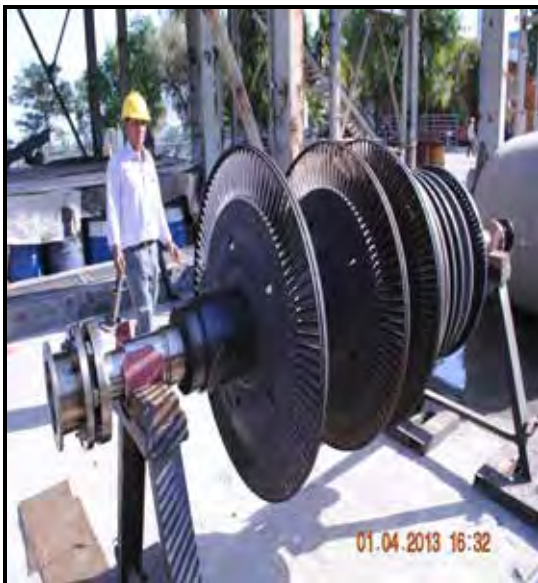
101-JT ROTOR BEFORE CLEANING
