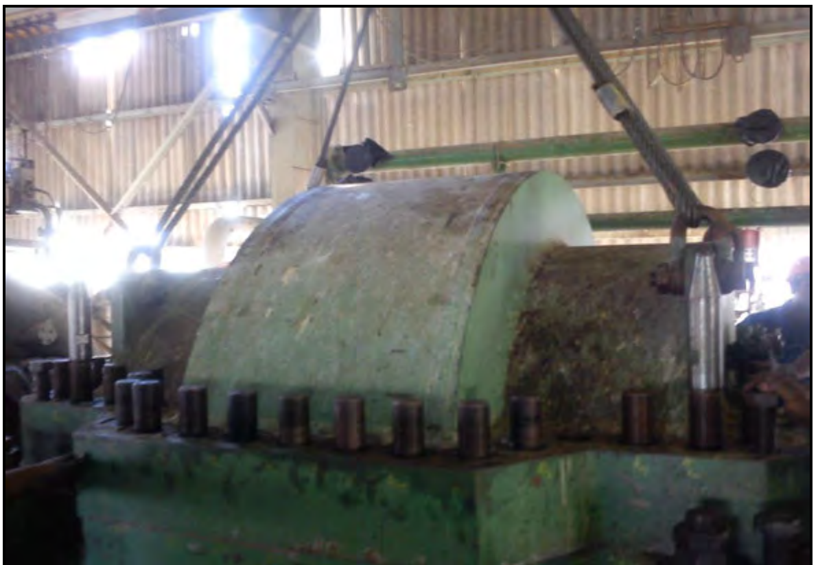
Lifting arrangement of top casing of LP case -1
