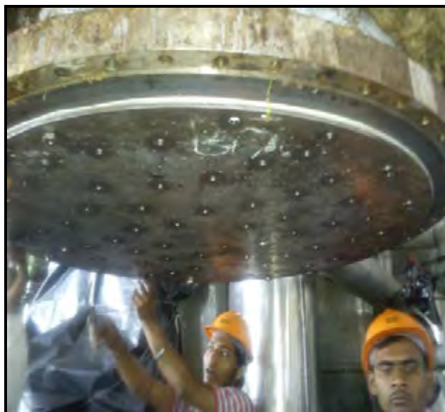
Assembly of perforated plate with Teflon sheet
