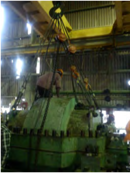
Lifting arrangement of top casing of LP case - 2
