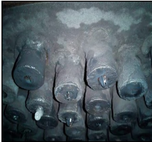
Orifice plugs in bottom tube sheet
