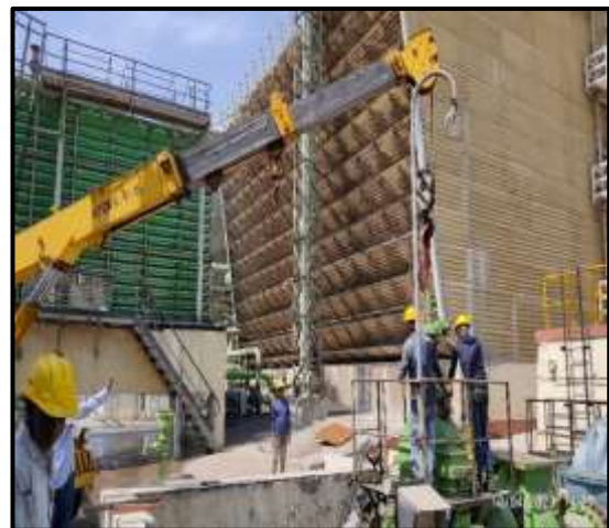
NRV and Gate valves repairing
