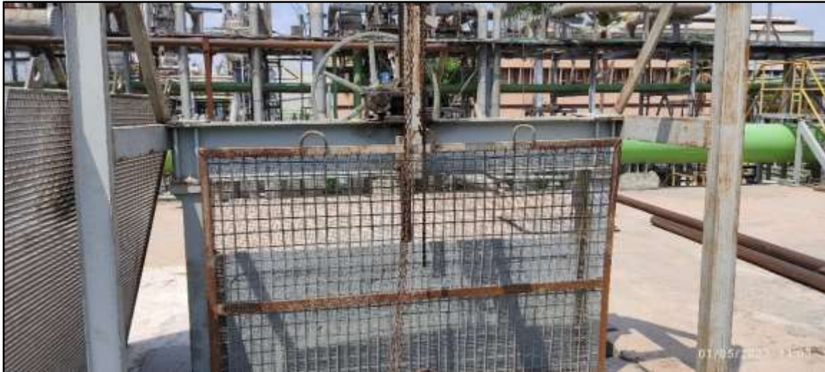
Jash make Sluice Gates preventive maintenance
