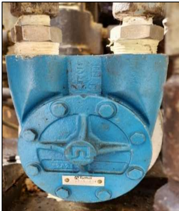
New AOP with motor of tuthill make was installed
