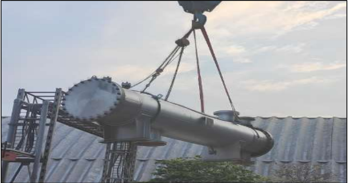
Lifting of new heat exchanger
