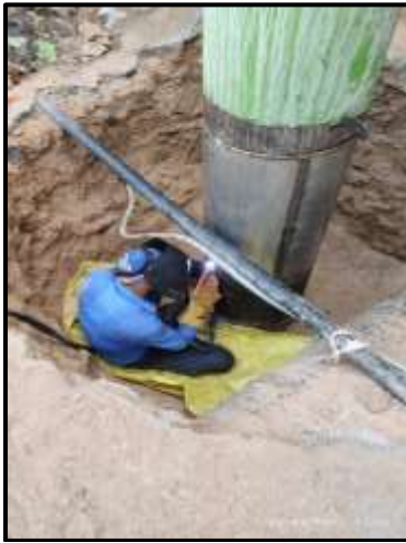
SS-304 plate cladding work with subsequent wrapping coating
