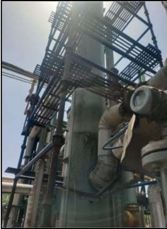
K-1 Vessel in PGR Before coating
