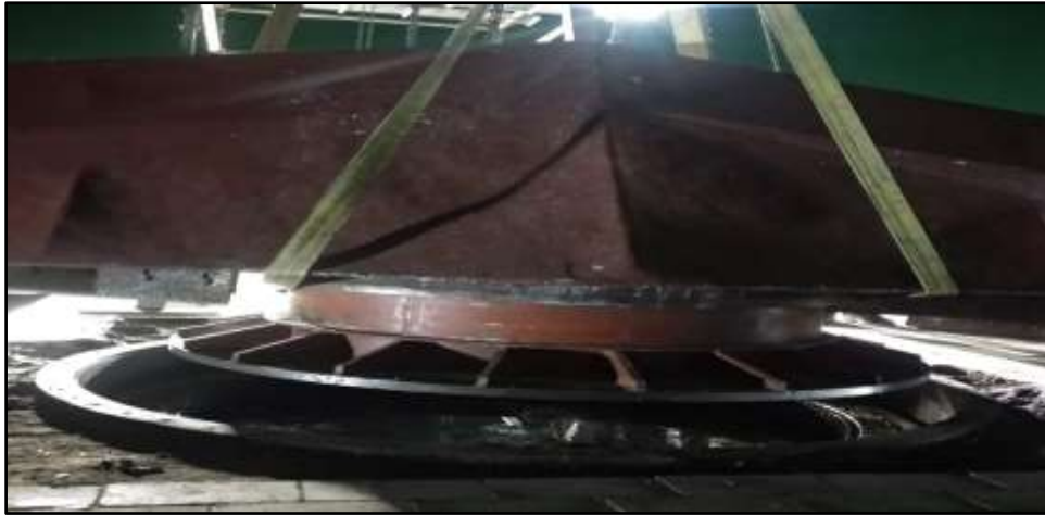
Scrapper arm lifted from position.
