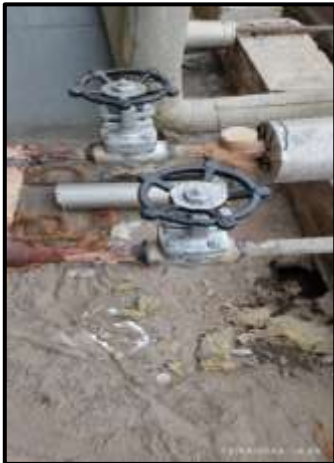
Gate valves replaced
