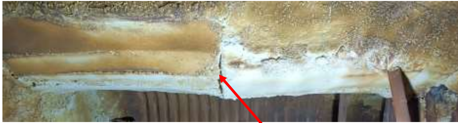
Damaged Refractory
