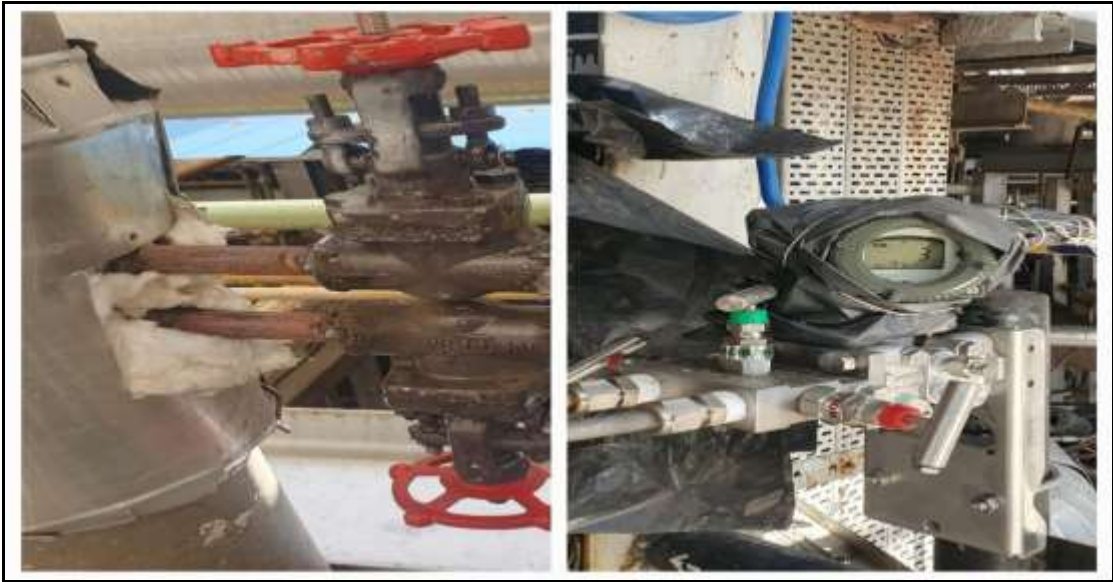
Fig – Orifice and isolation valves
