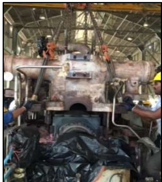
Lifting of Top casing
