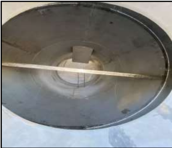
Inside view of new 103-F from top nozzle
