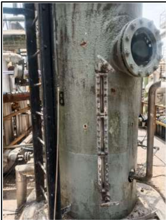
Bottom portion of B3A Vessel in PGR before Coating
