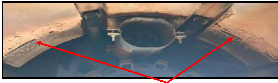
Damaged Refractory
