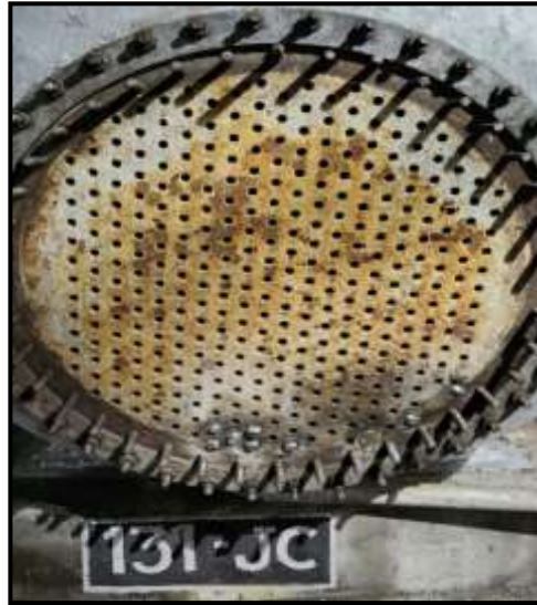
9 nos. tubes plugged (1 no. leaky & 8 nos. badly choked) in 131-JC
