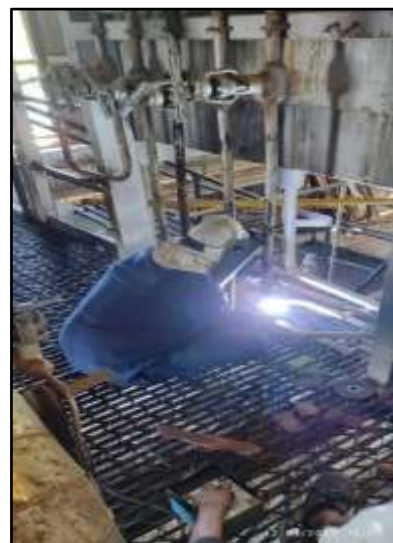
Vent lines repairing
