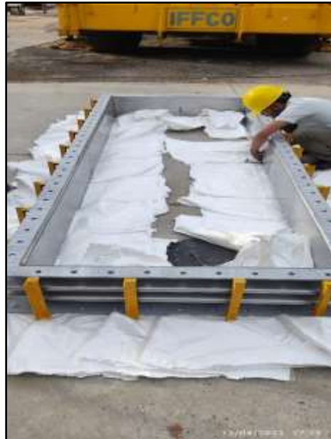
New Bellows for FD Fan Turbine duct
