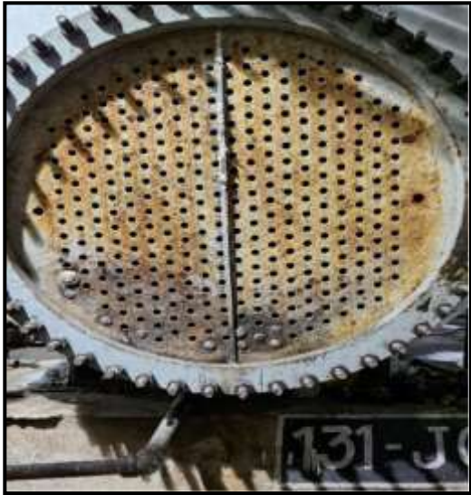
9 nos. tubes plugged (1 no. leaky & 8 nos. badly choked) in 131-JC
