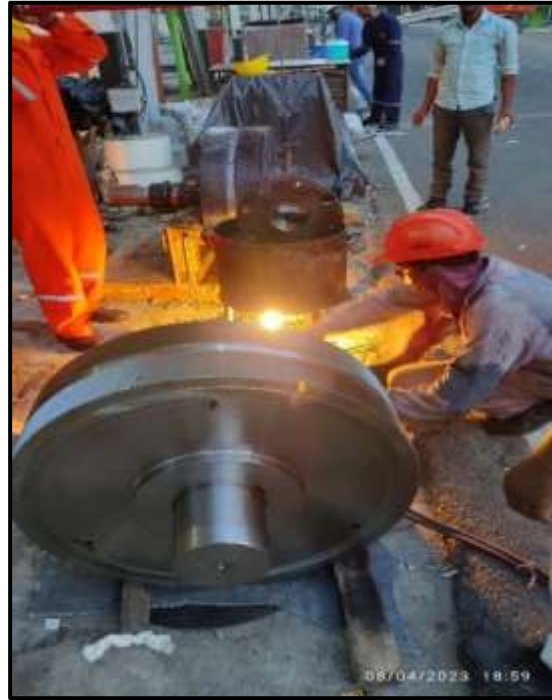
New gear wheel for Q-4411
