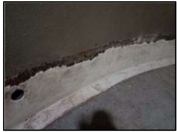
Surface prepared by grinding
