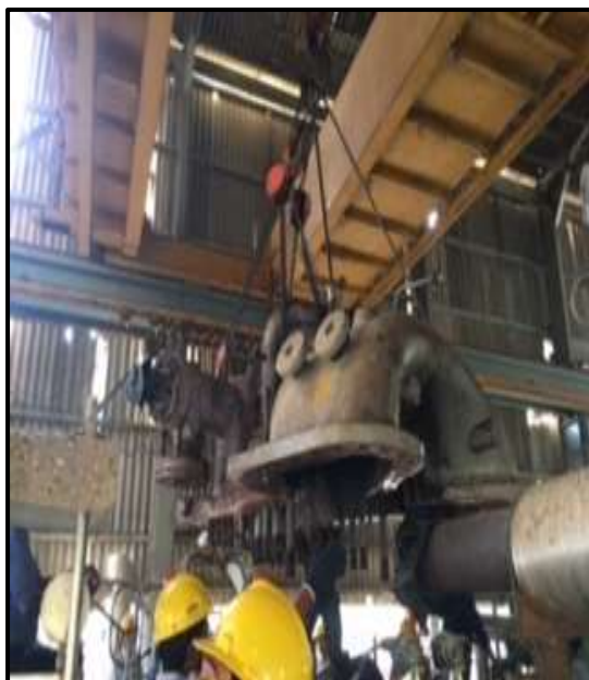
Removal of Top casing of turbine
