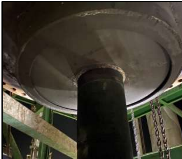
Weld fillup done on eroded welding
