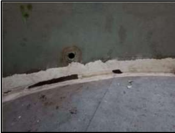
Coating peeled off at many location inside DM Water Tank
