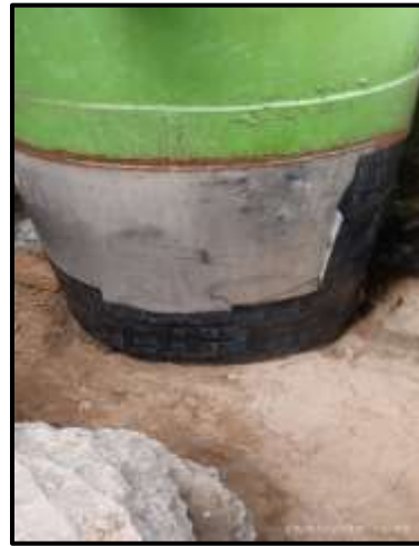
SS-304 plate cladding work with subsequent wrapping coating
