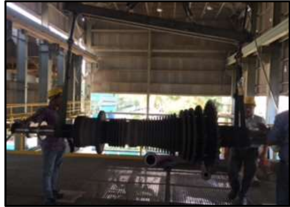
Rotor shifting to stand
