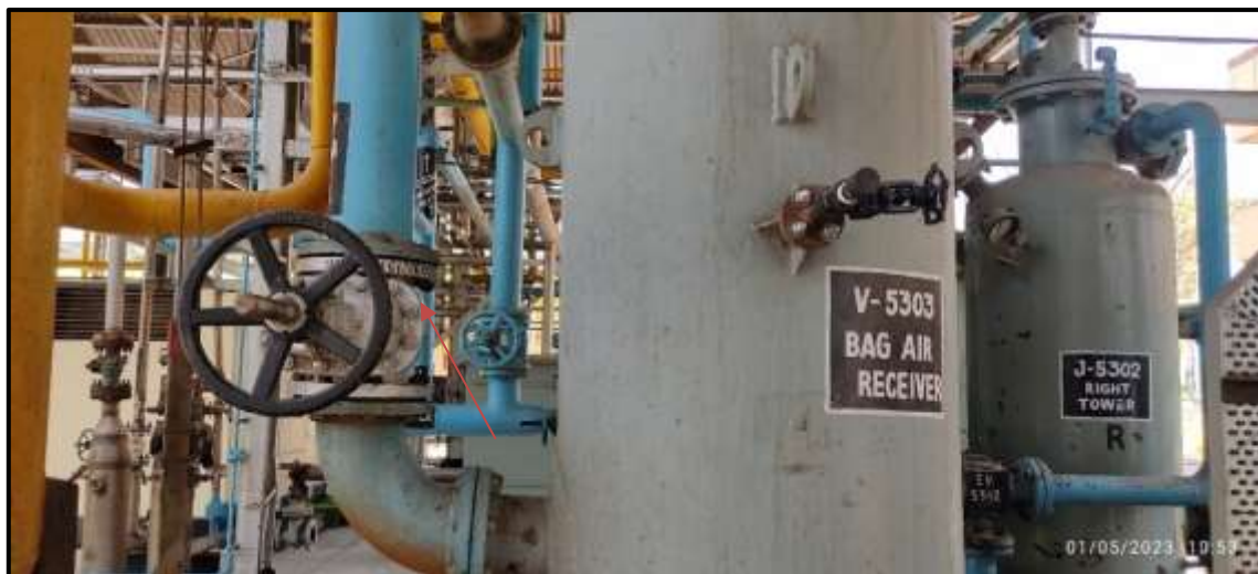
6" X 150# Gate valve replaced
