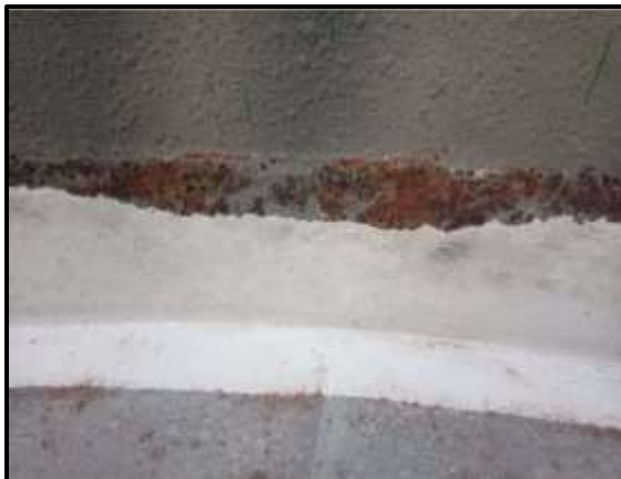
Surface prepared by grinding
