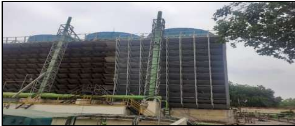
Erection and commissioning of cell No. 3 of NCT
