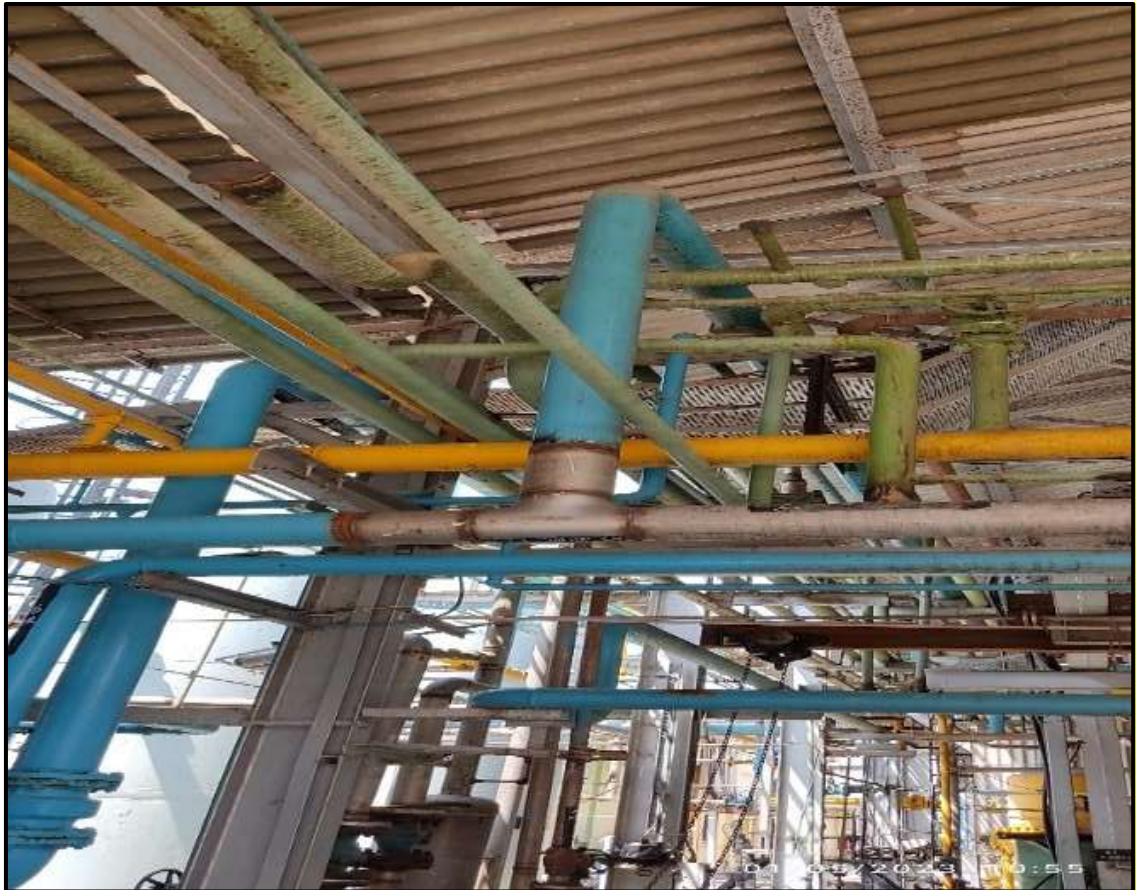
Redundant Cooling water lines removal
