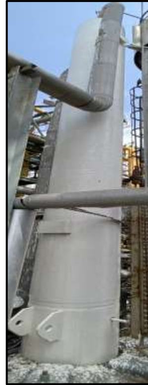
K-1 Vessel in PGR After Coating
