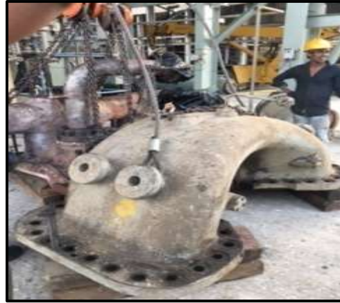
Top cover placed over slippers
