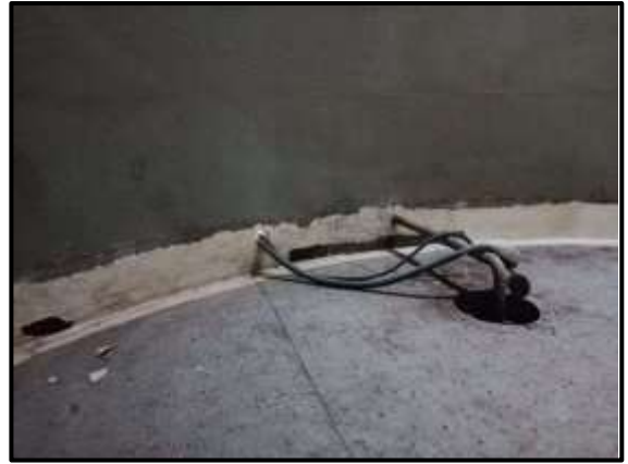
Coating peeled off at many location inside DM Water Tank
