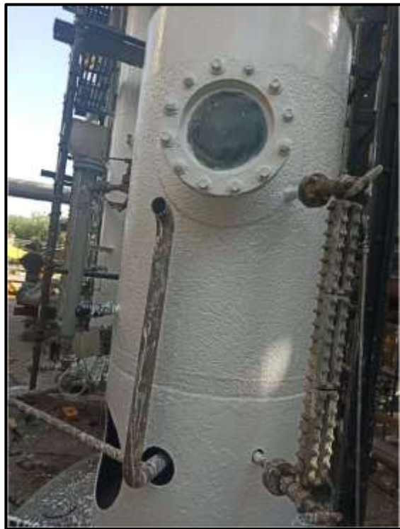
Bottom portion of B3A Vessel in PGR after Coating
