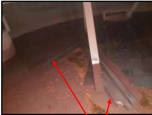
Tray Segment laying on bottom DE
