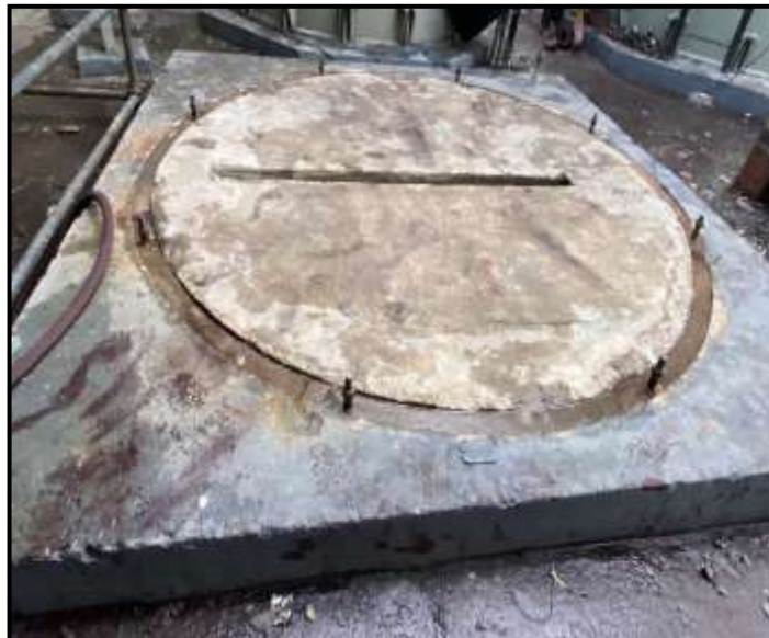
Foundation after removal of 103-F
