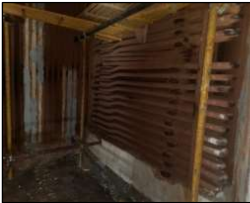
Refractory inside boiler furnace
