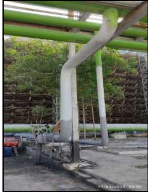
Zinc coating on cooling water pipelines
