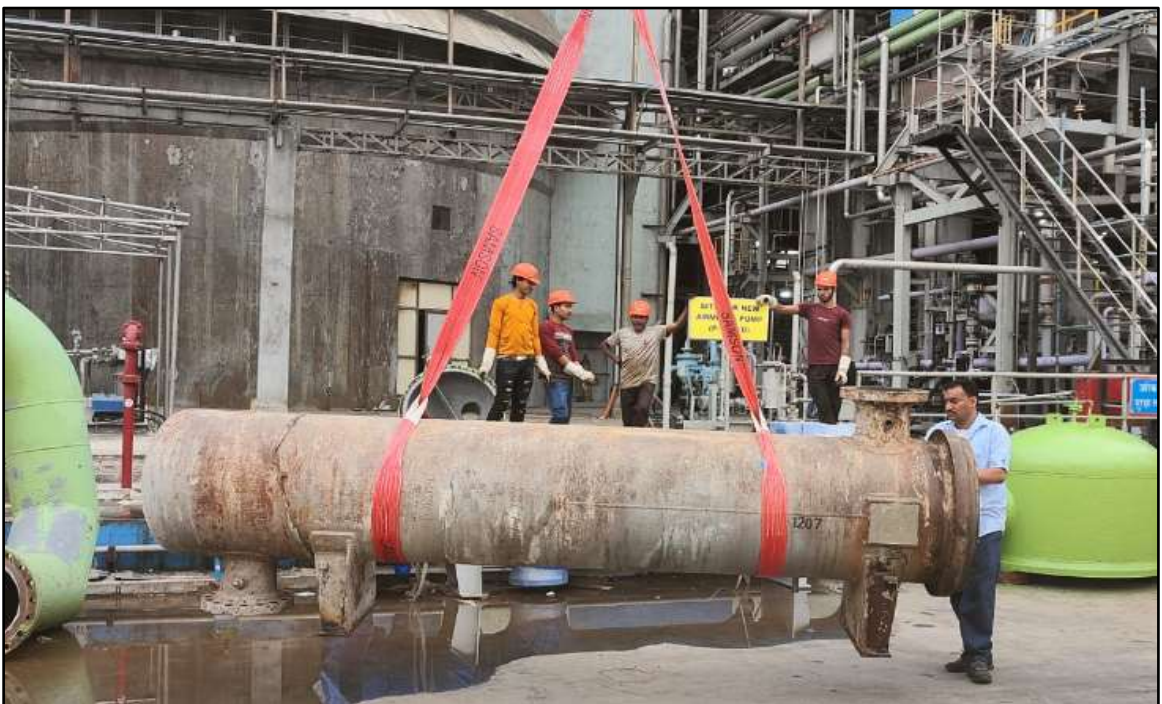
Old heat exchanger being removed.
