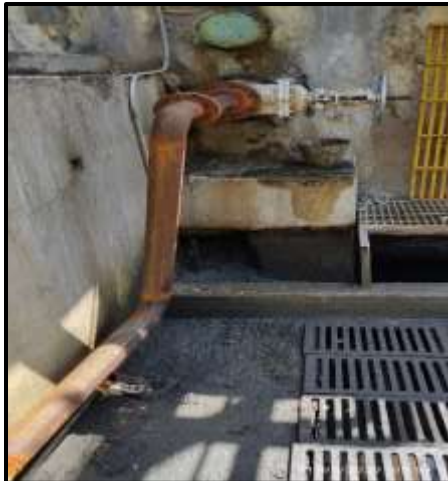
Old urea basin drain line replacement
