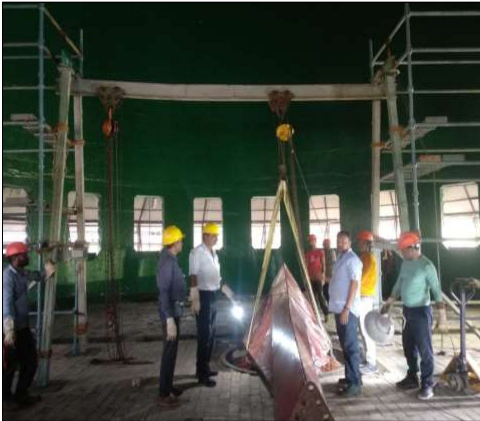
Derrick arrangement for removal of scrapper arm.
