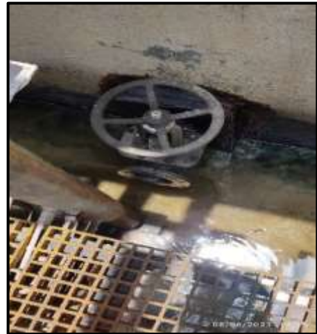
Basin drain line valve replacement
