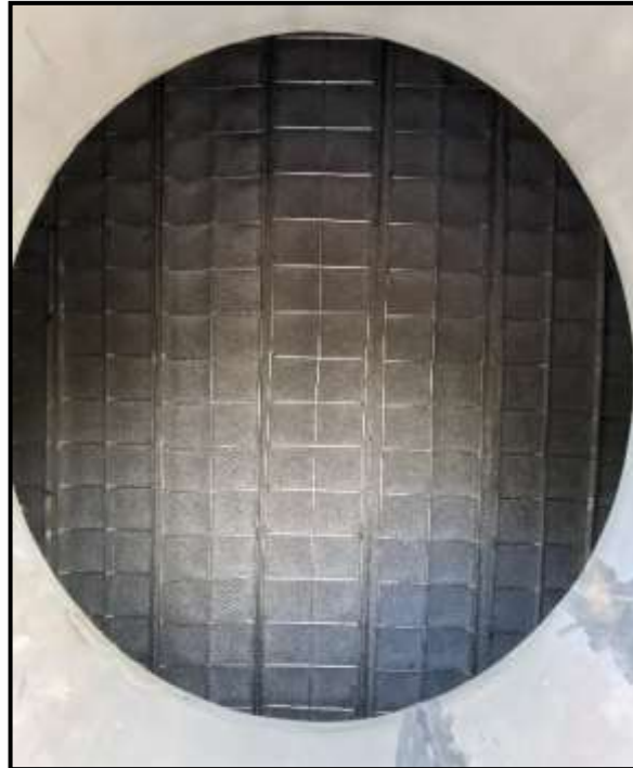
Demister Pads installed
