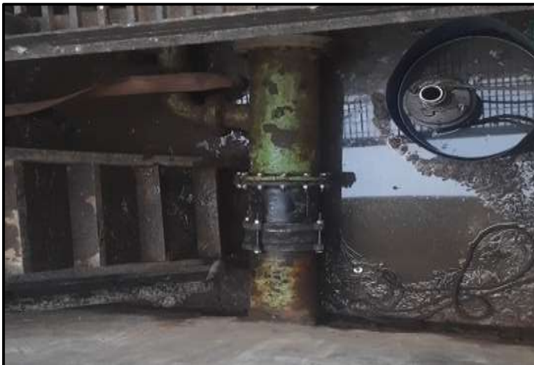
New CID spigot joint
