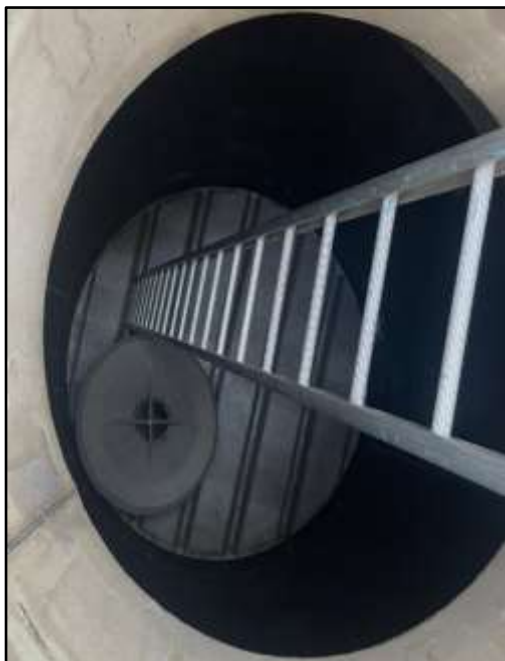
Top manhole removed
