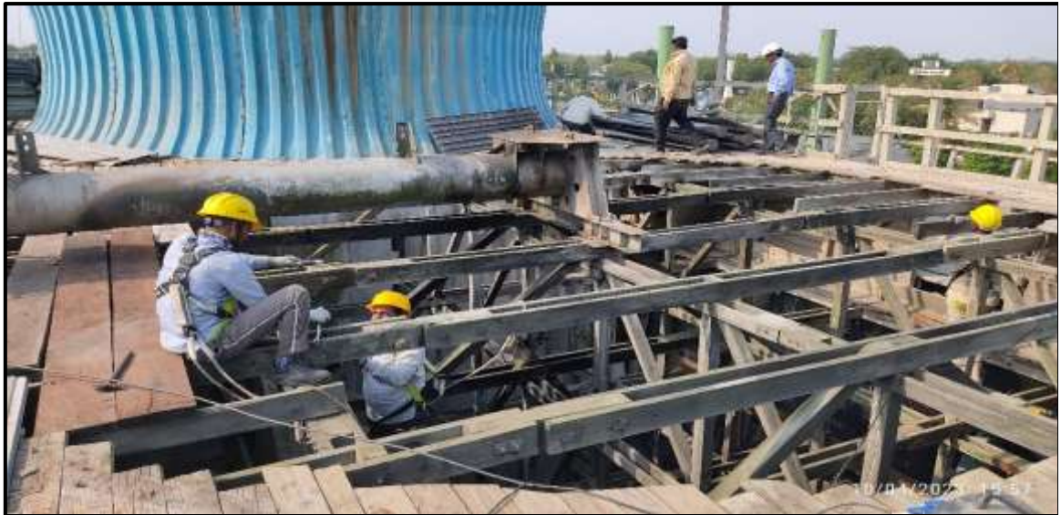
Damaged timber replacement work
