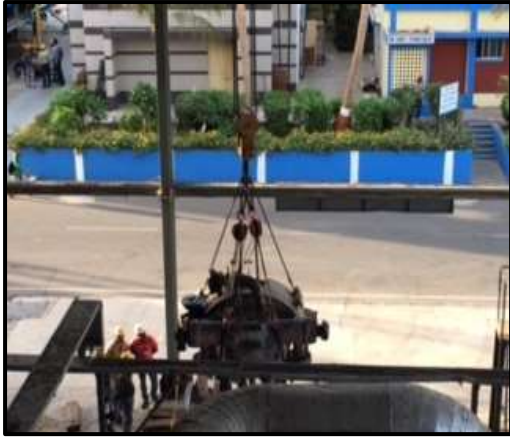
Shifting of Top casing cover
