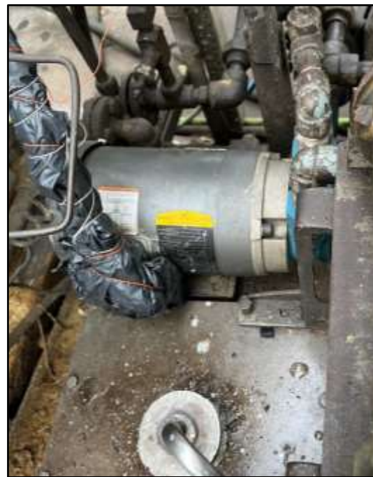
New AOP with motor of tuthill make was installed
