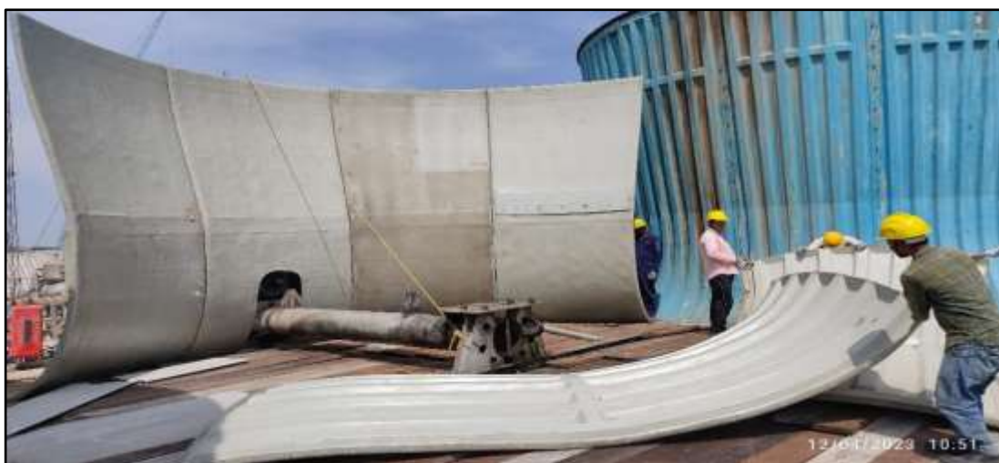
Cooling Tower Cylinder, Fan Blade and Hub assembly replacement
