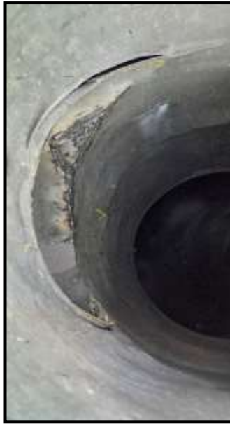
Weld Repaired Liner
