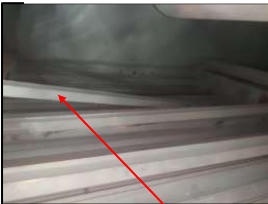
Tray Segments found dislocated from its position
