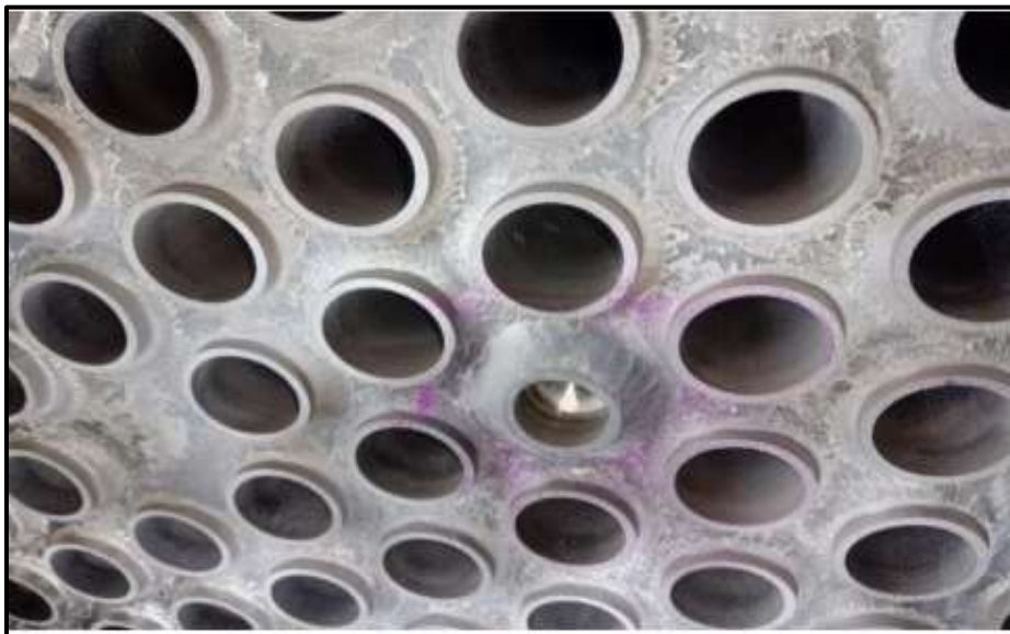
Bottom tube sheet side tube plug
