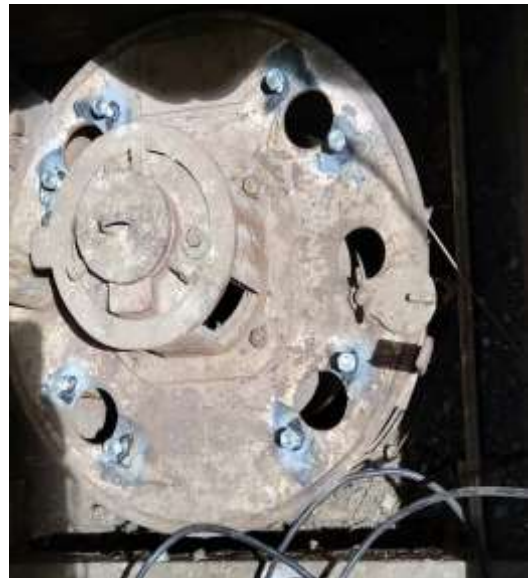
Arch burners new studs welded
