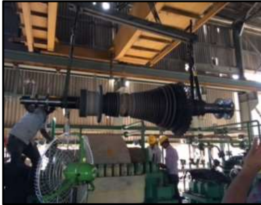
Lifting of Rotor under progress
