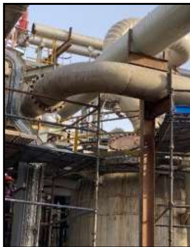
Pipe Supports erected & cut the lines
