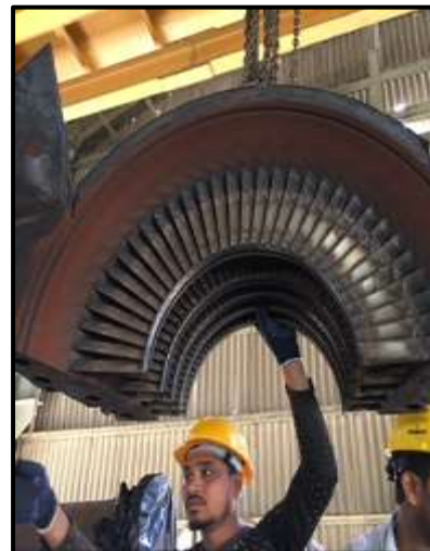
Diaphragm assembly lifted
