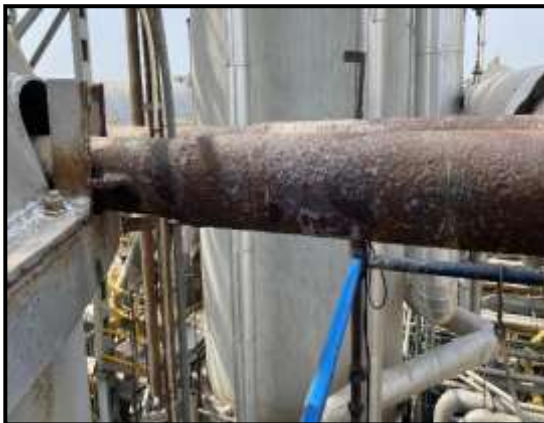
Corroded pipe pieces of start-up heater outlet line
