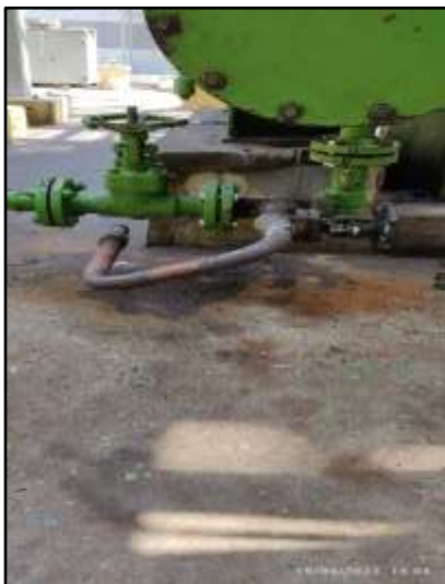
Cooling water drain line extension work
