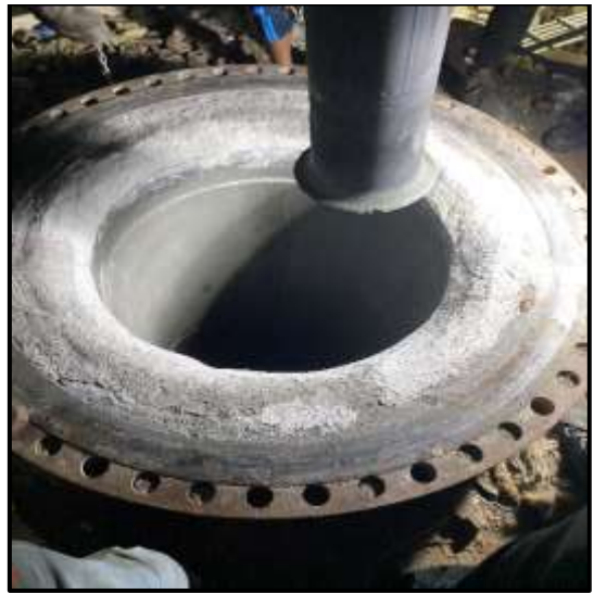
Top Flange Refractory repaired
