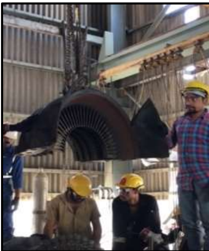
Removal of diaphragm assembly
