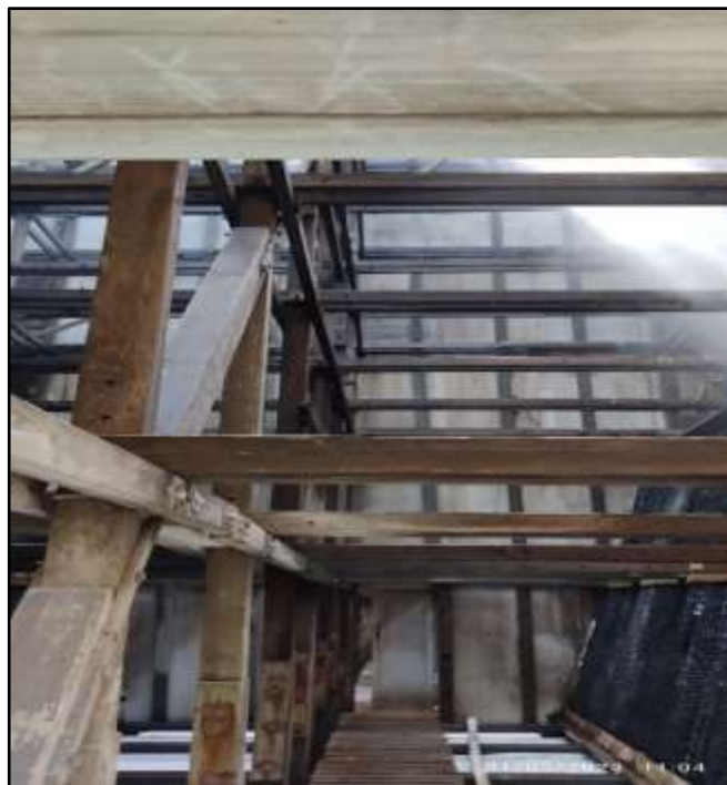
Partition wall rearrangement work
