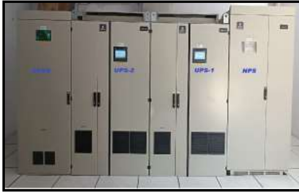
Vertiv UPS Model: Liebert FP60Z with SCVS and NPS
