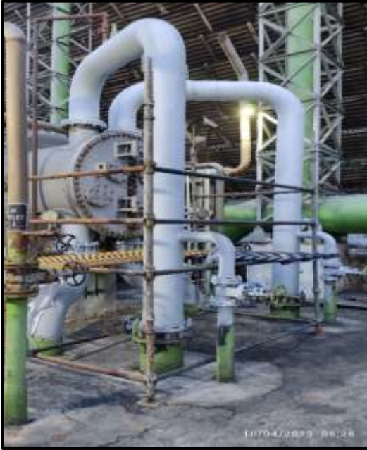
Zinc coating on cooling water pipelines
