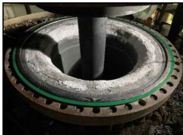
Box-up of Top cover with new gasket
