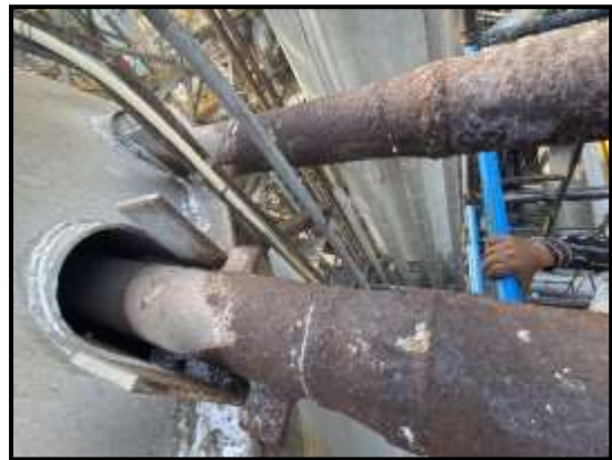
Corroded pipe pieces of start-up heater outlet line
