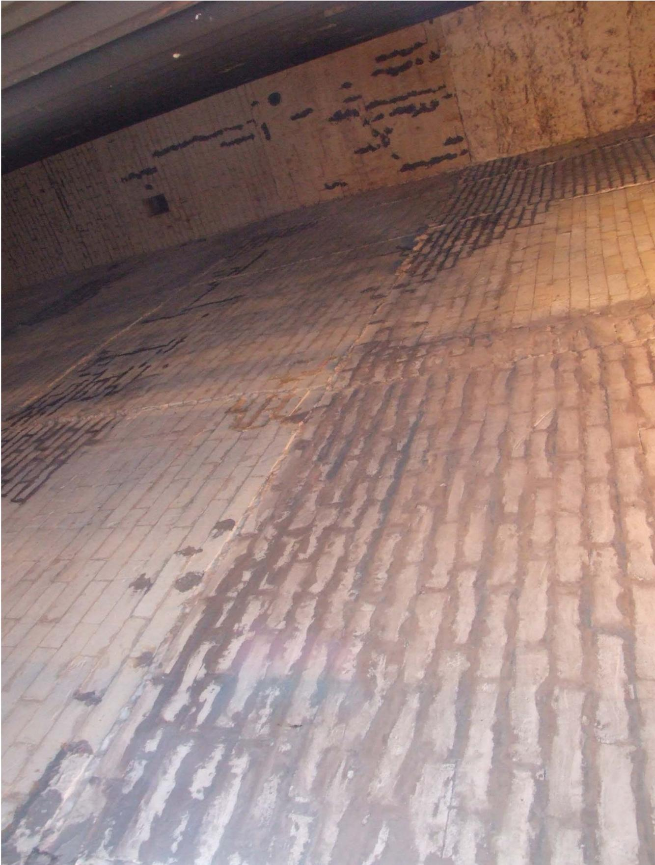
LINING OF RADIANT SECTION OF PRIMARY REFORMER
