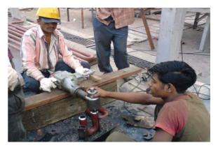
Fig. 18 Edge preparation by Machine tool
