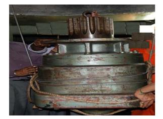
Gearbox is being removed from bottom
