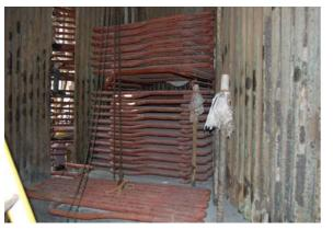
Fig. 11 Cut Spacer tubes S2 & S4 No any bank tube on PSH opening
