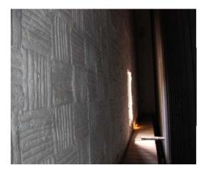
CF Module Insulation on Wall No 3
