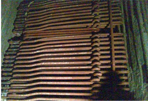
**Fig.13 PSH Coils After Work**
