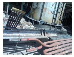
Fig. 16 Template made for Coil Repairing
