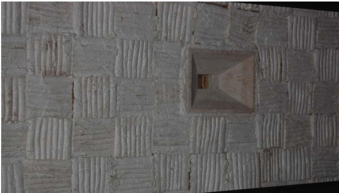
Ceramic Fibre Module Insulation on Wall No 4
