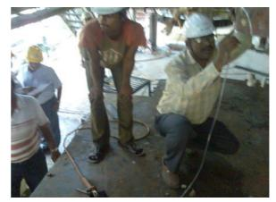
Fig. 8 Transfer of Vertical Dimension by Water Level PVC Tube
