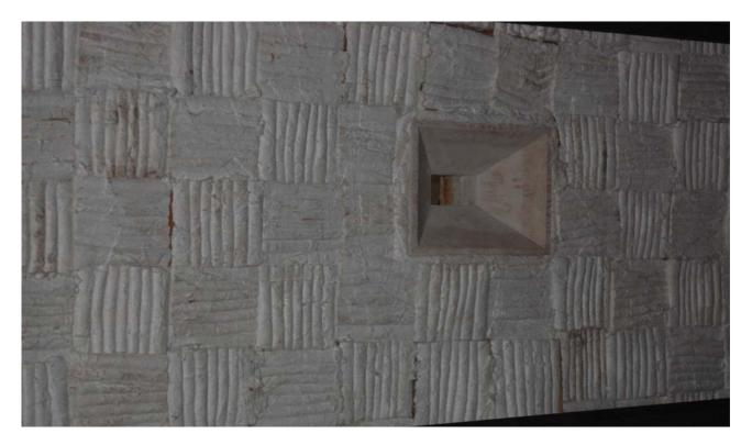
**Ceramic Fibre Module Insulation on Wall No 4**
