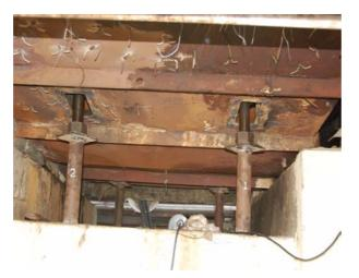
Fig. 27 Arrangement made for Bearing Removal
