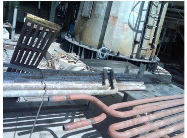
**Fig. 16 Template made for Coil Repairing**
