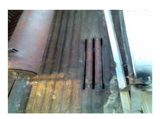
Fig. 21 Location of Furnace Rear Panel Tubes Cut for Insertion of PSH Coils in Furnace
