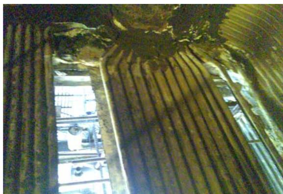
**Fig.12 View after removal of Refractory.**
