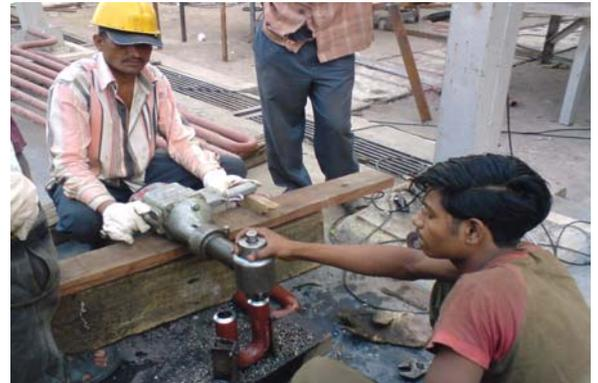
**Fig. 18 Edge preparation by Machine tool**
