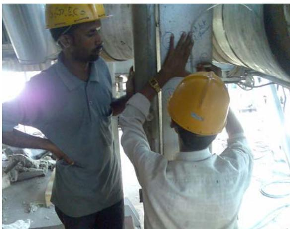
**Fig. 9 Level marking on Column**
