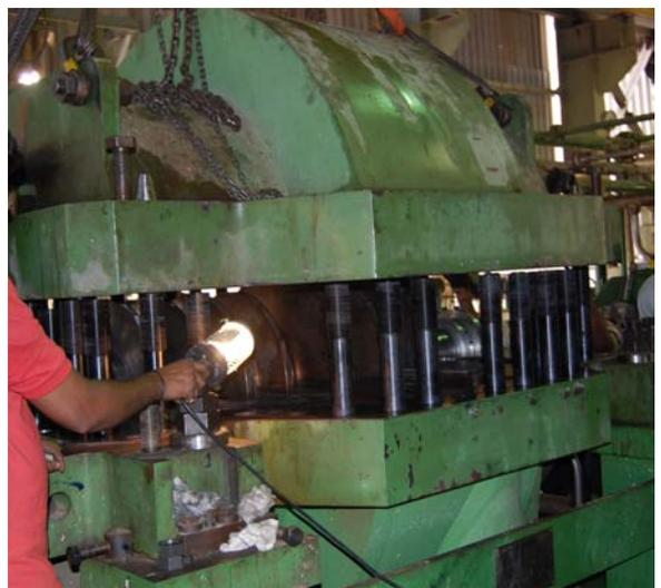
**Boxing up of top casing of LP Compressor**
