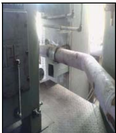
HP Ammonia Pump Discharge line support rectification
