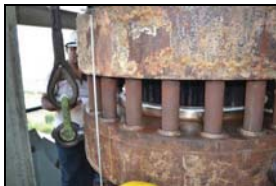
Lowering of tube bundle
