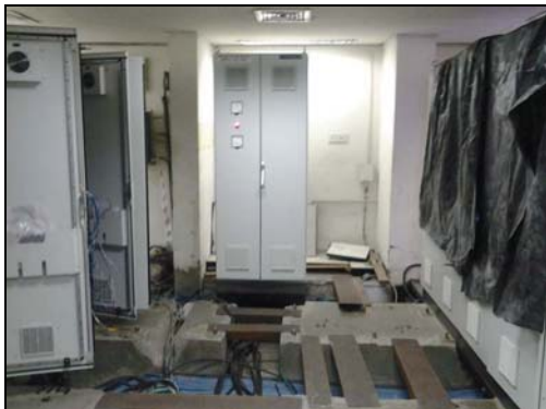
Replacement of DCS Marshalling Cabinets
