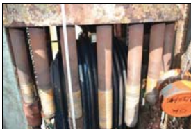
Lowering of tube bundle with help of 4 nos. of guide pipe -5
