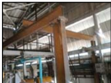
Beams erected for the easy removal and rigging of the burners
