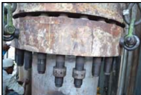
Bottom dome – after removing the nut except 4 nos. of loosened nut
