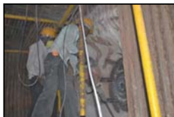
Breaking and removal of Burner Block refractory
