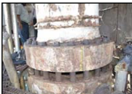
Lifting of top dome - 1
