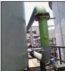
Installation of Orifice Flow Plates
