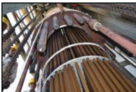
Lowering of tube bundle with help of 4 nos. of guide pipe -2
