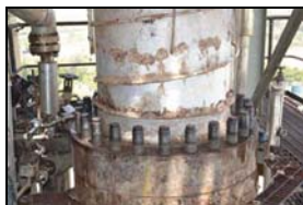
Top dome flange – after nut removal
