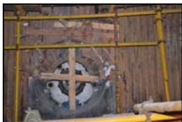
Casting of Burner Block refractory
