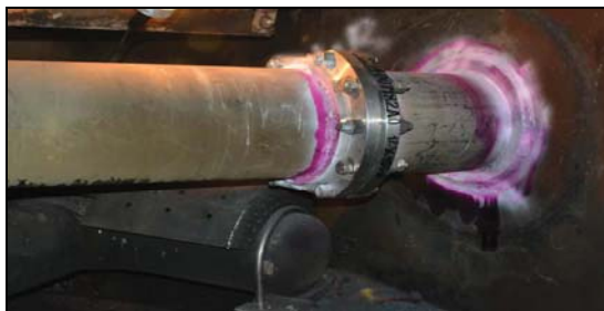
102-EB NEW INLET NOZZLE FROM INSIDE
