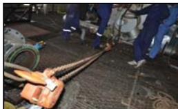
Removal of Burners from its position
