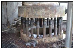
Lifting of top dome – up to stud
