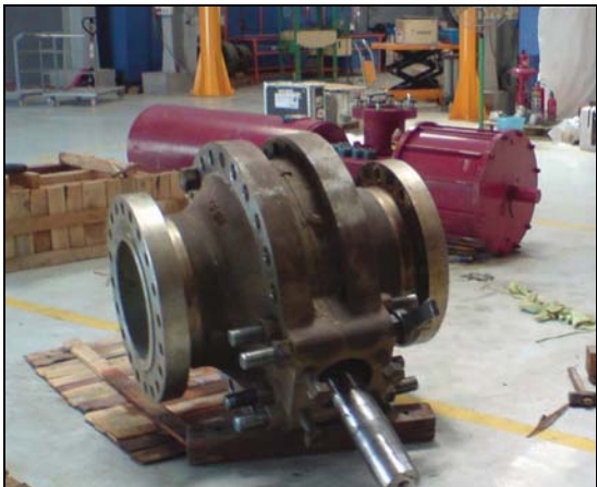
USV – 933 Control valve under dismantling
