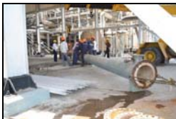
Pulling out of tube bundle of H-1813
