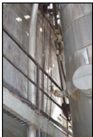
Rigging arrangement – North side
