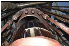
Lowering of tube bundle with help of 4 nos. of guide pipe -1
