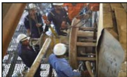
Removal of Burners from its position
