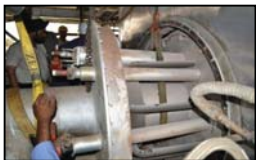
Removal of Burners from its position
