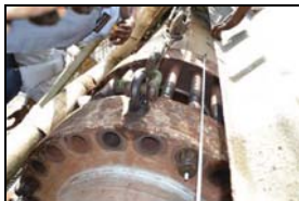
Lowering of tube bundle with help of 4 nos. of guide
