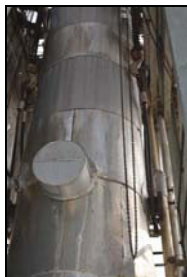
Rigging arrangement – South side
