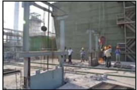
Removal of old Gates
