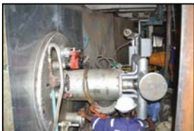
Installation of Burners after modification
