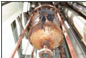
Lowering of tube bundle with help of 4 nos. of guide pipe -4
