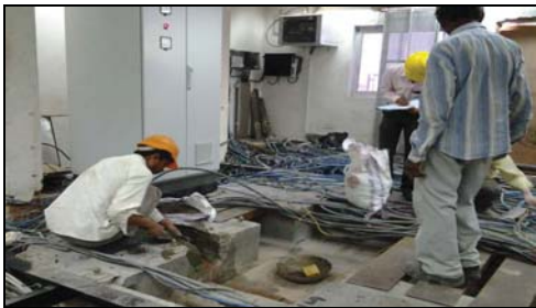
Widening and preparation of Cable trench inside DCS Marshalling Room
