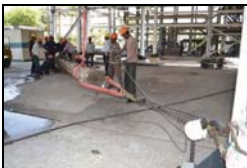
Pulling out of tube bundle of H-1813
