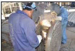
Cutting of tubes with the help of cut rods-1
