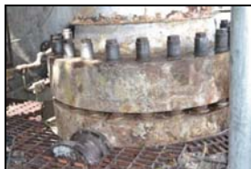
Lifting of top dome
