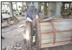
Cutting of tubes with the help of cut rods - 2
