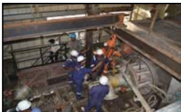
Removal of Burners from its position
