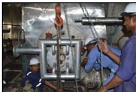
Installation of Burners after modification
