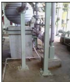
HP Ammonia Pump Discharge line support rectification
