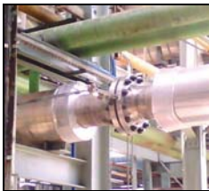
Installation of FI-14 in 116-JA/JB pump discharge line
