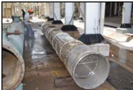
Hydrojetting of H-1812
