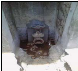
Drain at New CT cell no. 3.
