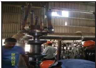
4 ata control valve – removal of stem
