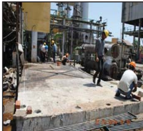
Photographs showing new foundation and cores.
