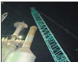
Removal of Pressure shell
