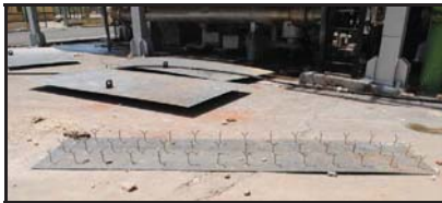
NEW Y-TYPE ANCHOR WELDED ON NEW MS PLATE
