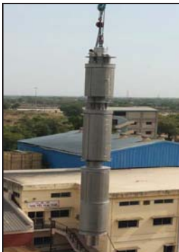
Top portion of inner collector lifted
