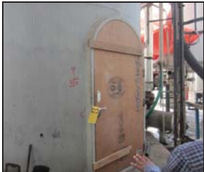
A wooden door was made to cover the opening of skirt
