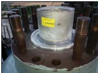
Special gasket welded with outlet insulation sleeve and top insulation sleeve welded with outlet insulation sleeve
