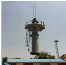
Pressure shell lifted
