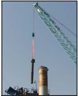
Removal of Inner collector 2 nd piece
