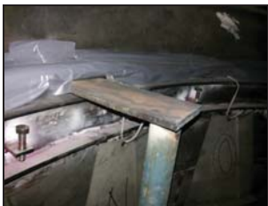
At outer end it was supported at 4 th bed outer collector
