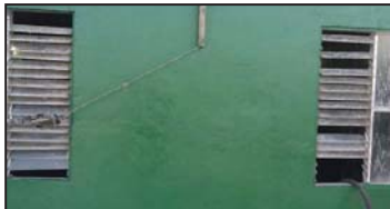
Prill Bucket room walls with Greensboro treatment
