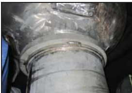
Sleeve positioned and tack weld done.
