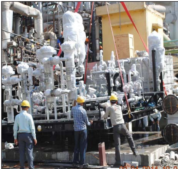
NEW SYSTEM BEING ERECTED ON FOUNDATION
