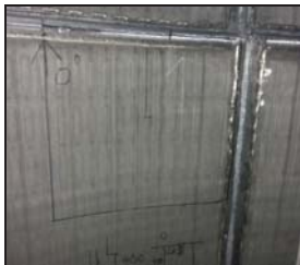
Marking for cutting of mesh and perforated plates below existing rings
