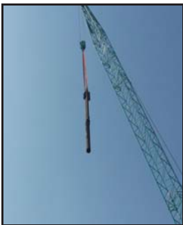
Removal of inner collector 3 rd piece
