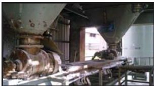
Modification in V-1702-2/3 : additional flange provided
