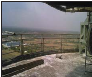
New SS 304 prill tower top railing
