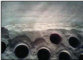
DP CHECK AFTER FINAL WELDING
