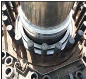
122-C after completion of seal welding
