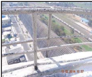
Existing MS prill tower top railing
