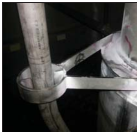
Sliding support of AT thermowell pipe
