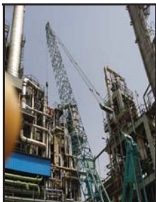
Removal of old LPCC (1)
