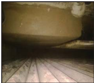
NEW REFRACTORY 165 MM THICK AS SHOWN IN SKETCH
