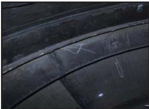
1 st bed outer collector
