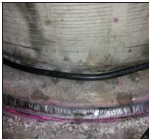
After full welding
