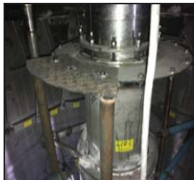
At centre scaffolding was bolted with stuffing box ring plate
