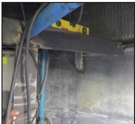
Additional support structure was made by providing channels
