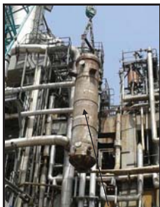
Removal of old LPCC (4)
