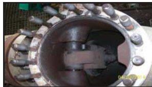
23 ata check valve – removed top cover
