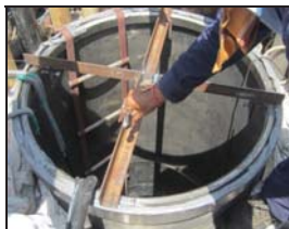
Piano wire was dropped from top Pressure shell flange
