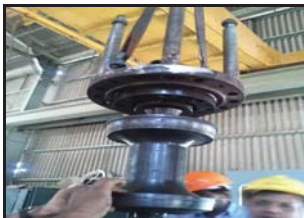
4 ata control valve – removal of stem
