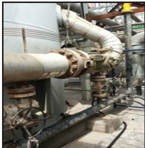
Rupture disc was dropped and line was provided
