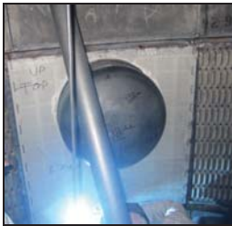
Installation of first panel
