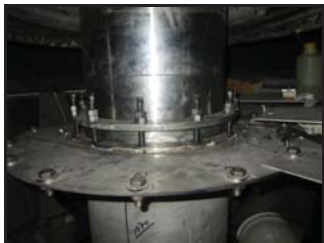
Stuffing box after installation of packing
