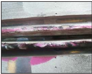
Lip seal joint area after cutting
