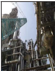
Erection of new LPCC (1)
