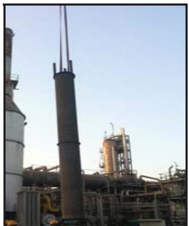
Removal of 4 th bed Inner collector
