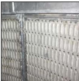
Perforated plates of 1 st bed after removal of wire mesh
