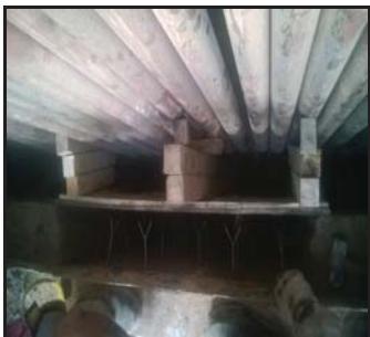
SHUTTERING ARRANGEMENT
