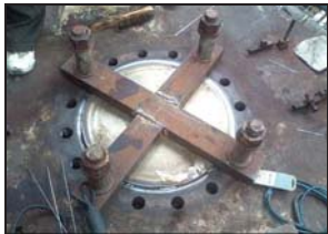
ARRANGEMENT MADE FOR TACK WELD DIAPHRAGM
