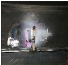
Clit was welded on protection screen support ring and supported with basket shell
