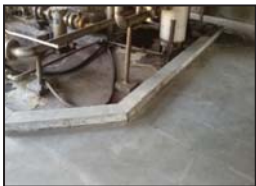
Bagging silo screen and transfer tower area after application of Kota Stones.
