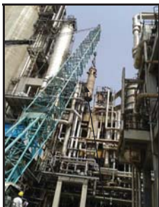
Removal of old LPCC (3)
