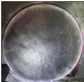
Old manhole at 3rd bed bottom
