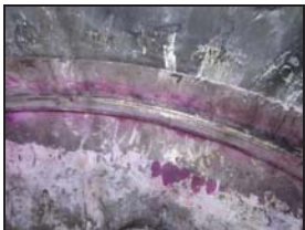
4 th bed bottom support ring after completion of welding
