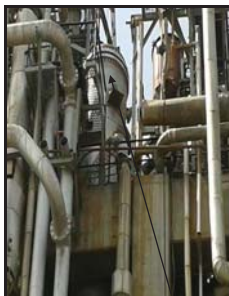
Erection of new LPCC (2)
