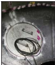
New manhole at 1 st bed bottom
