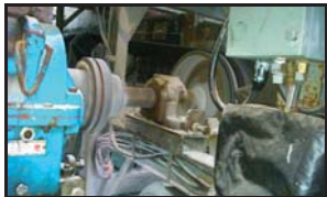
Pin-bush coupling from ingeco make gear box to head pulley
