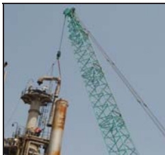
Removal of gas outlet line
