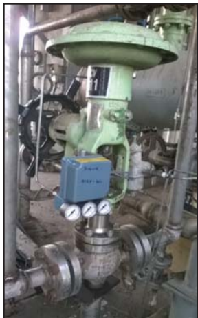
Eckardt makes valve positioner on HICV-1211 & LICV-1203
