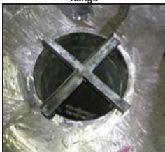
Fixture at 4 th bed bottom for adjusting piano wire
