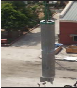
4 th bed inner collector lifted
