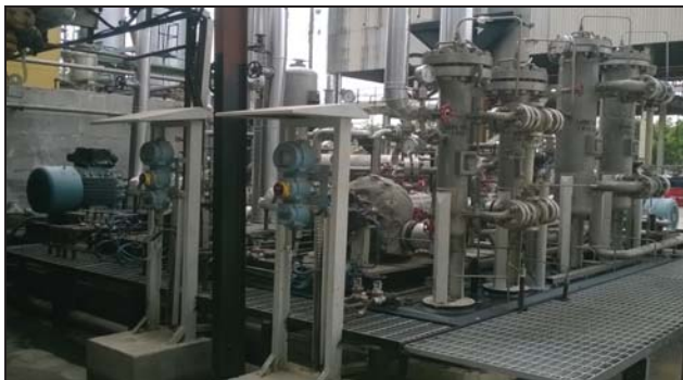
NEW 103-J LUBE OIL / SEAL OIL SYSTEM
