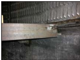
Additional support structure was made by providing channels
