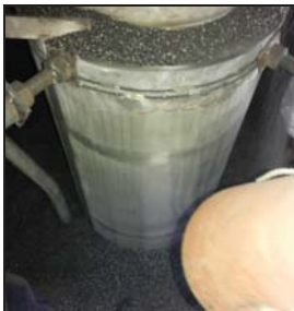
Catalyst filled below temporary scaffolding
