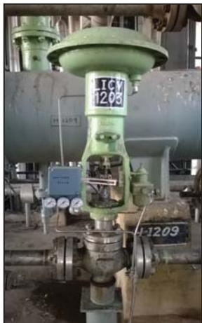
Eckardt makes valve positioner on HICV-1211 & LICV-1203
