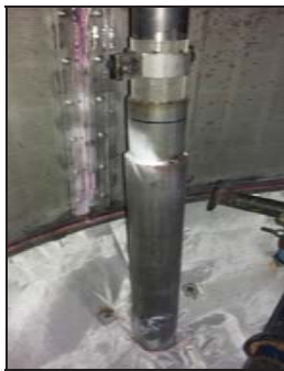
Bottom support of BT thermowell pipe
