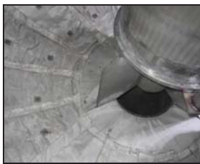
4 th bed bottom after providing insulation
