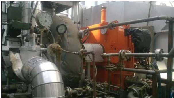
NEW ERECTED ID FAN DRIVE TURBINE & GEAR BOX
