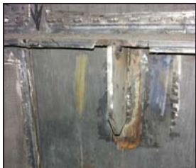
Temporary support provided at bottom of existing outer collector support ring
