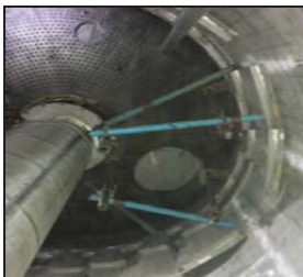
View of hanging scaffolding from 4 th bed bottom
