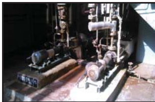
New base frame of P-1701 A/B
