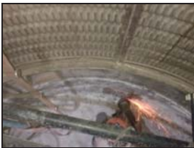
Removal of nitriding layer by grinding
