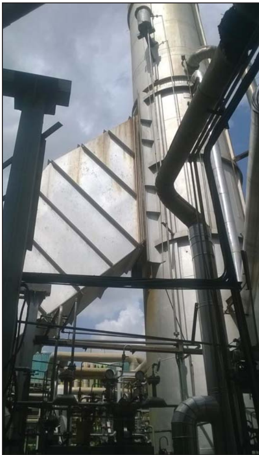
PROVISION OF OVERHEAD RUNDOWN TANK
