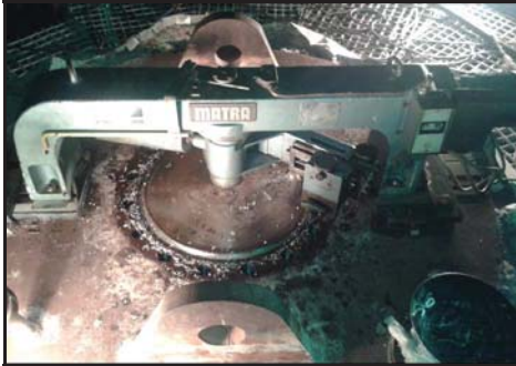
DIAPHRAGM CUTTING USING MATRA MACHINE
