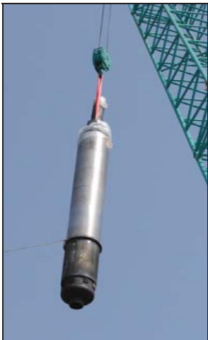
Removal of 122-C
