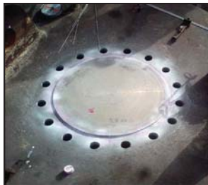
DP CHECK OF FINAL WELDING
