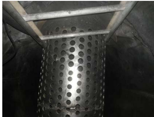
New Distributor welded on position
