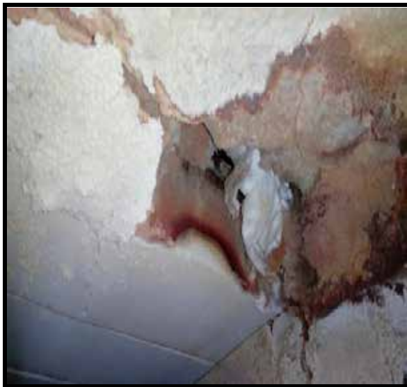
Location at which the tunnel block fallen in 4 th row
