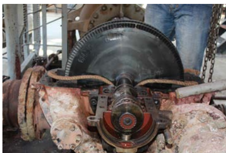
NDE side Bearing Pedestal
