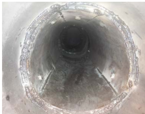
Repaired 103-D to 101-CA pipe Liner
