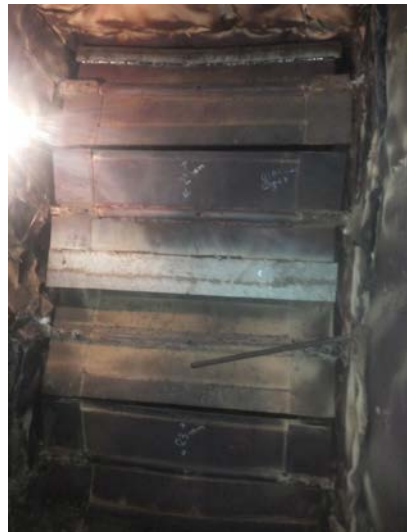
PRC-23 Dampers After Patch Plate Welding
