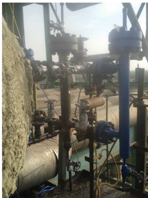
Assembly of Standpipe & Level Transmitter on Steam Drum
