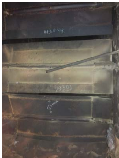
PRC-23 Dampers Before Patch Plate Welding
