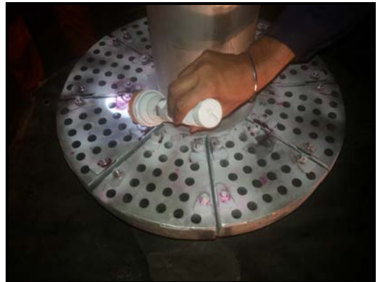
DP check of tack weld
