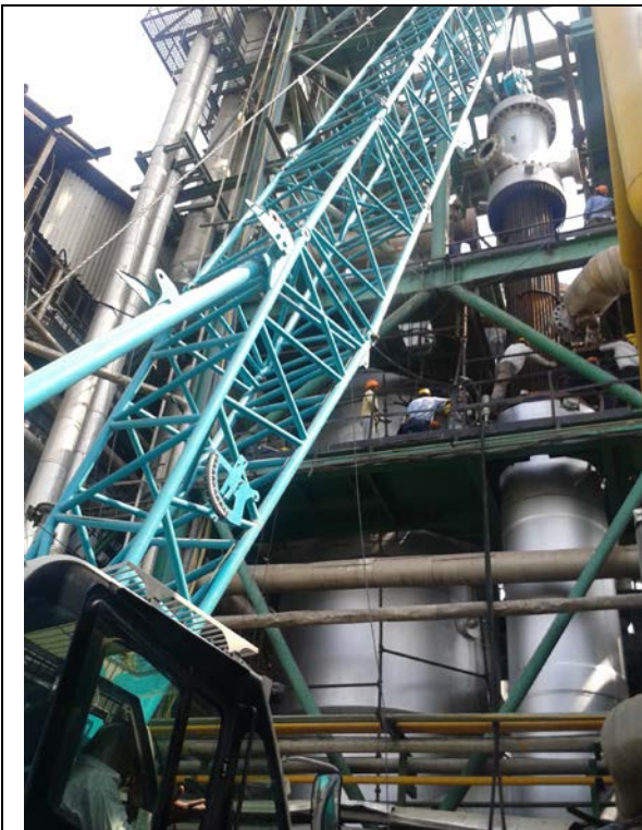
101-CB Tube Bundle Installation
