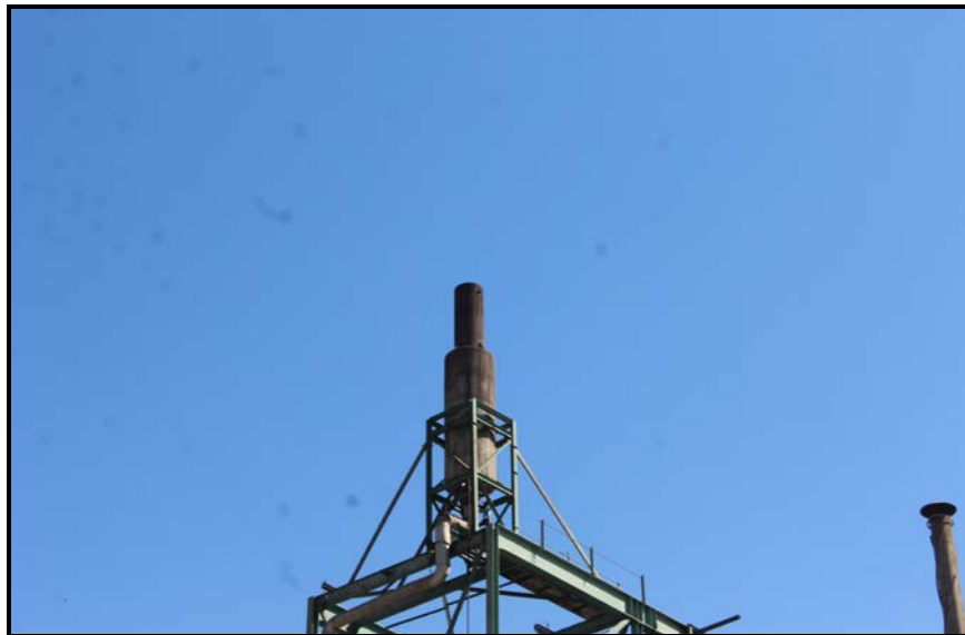
OLD SP-73 INSTALLED AT SITE
