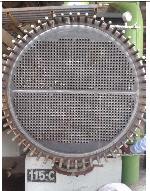
Tubesheet of 115-C after Seal Welding
