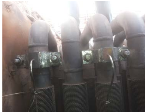
Clamp Installation on HT Superheat Coil
