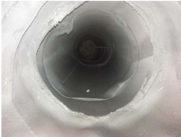
103-D to 101-CB pipe Liner
