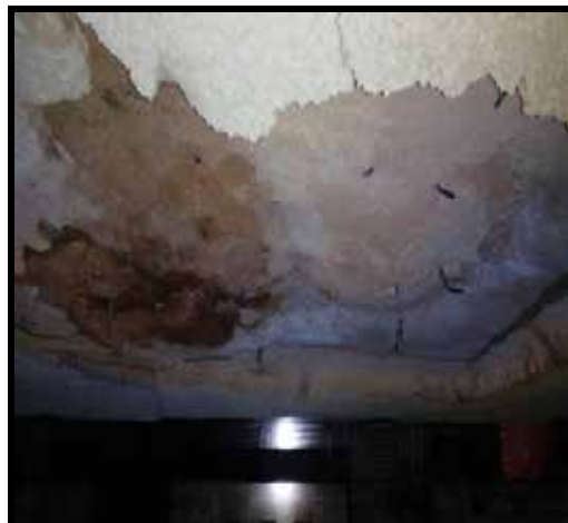
Ceiling Location from where the refractory dropped
