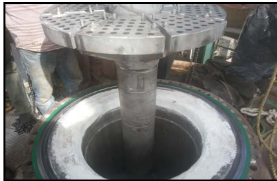
Refractory was repaired & setting of distribution grids
