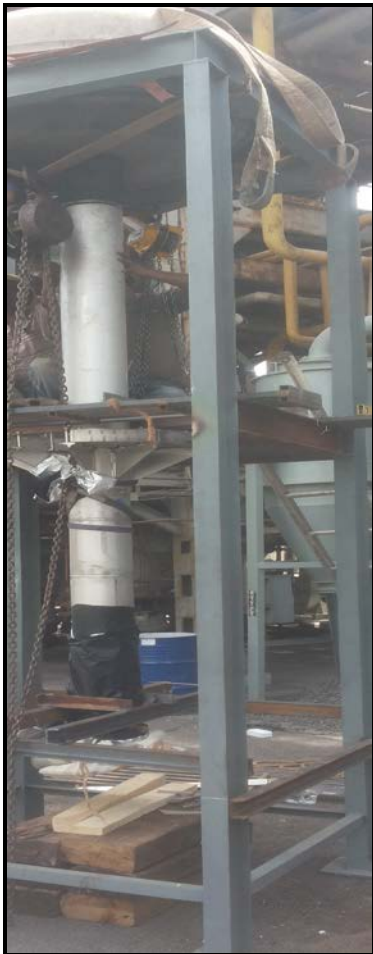
New Burner Pipe was set-up & welded on stand after confirming verticality
