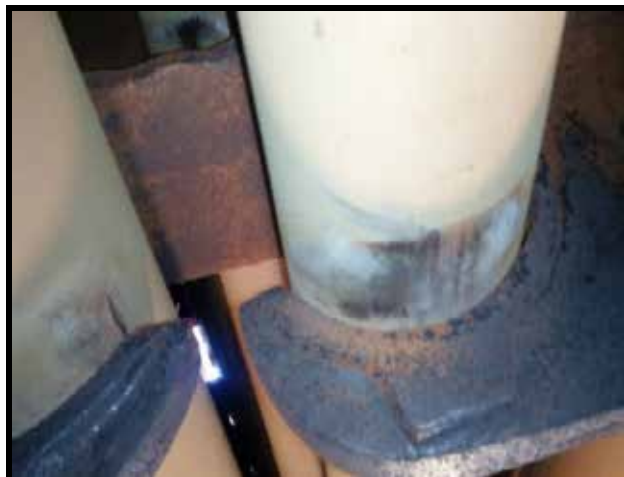
Rubbing marks on Coil bottom
