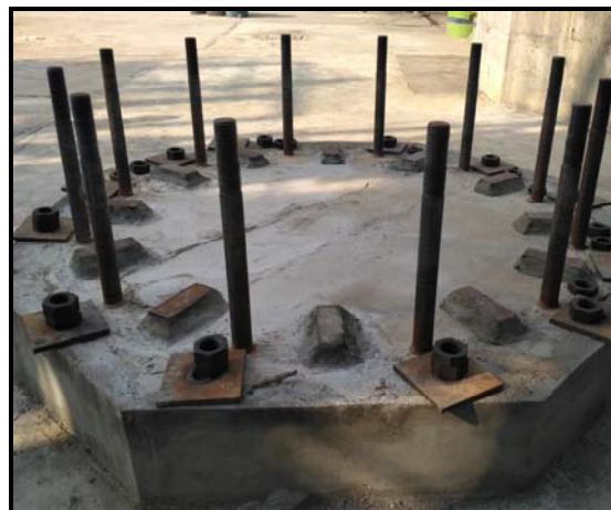
Template of 114-D in position
