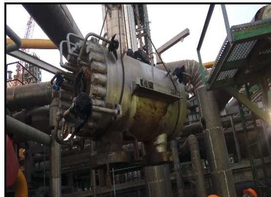
HP Case removed from foundation
