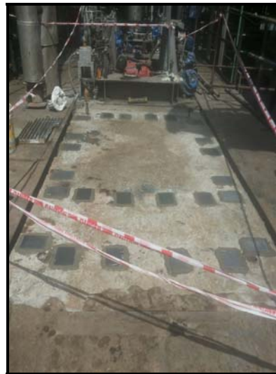
Packer plates fixed in their position using Shrinkomp
