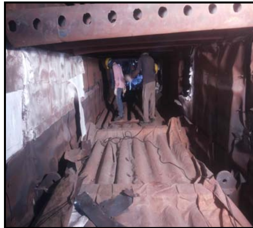
Old Steam Air coil removed from position
