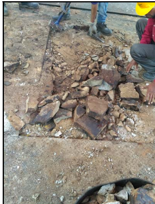
Breaking & removal of Old grouting matl.
