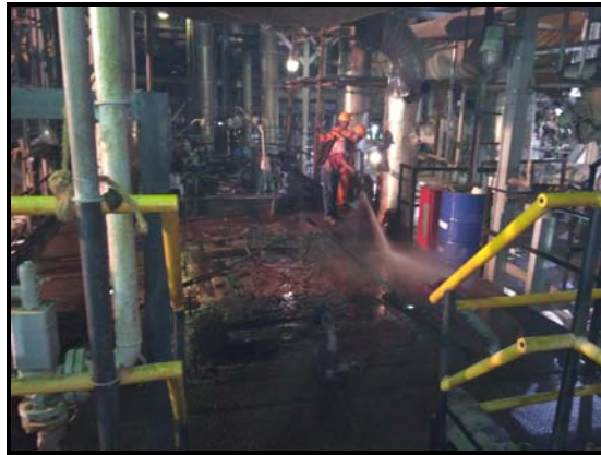
Turbine Floor Cleaning
