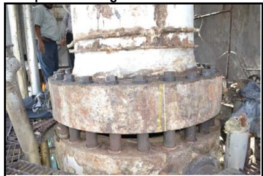
Lifting of top dome - 1
