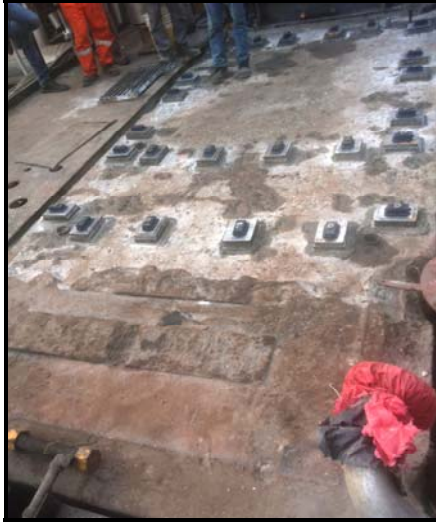
Foundation after positioning of shim plates and fixator
