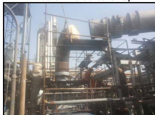
Exhaust line fabrication u/p
