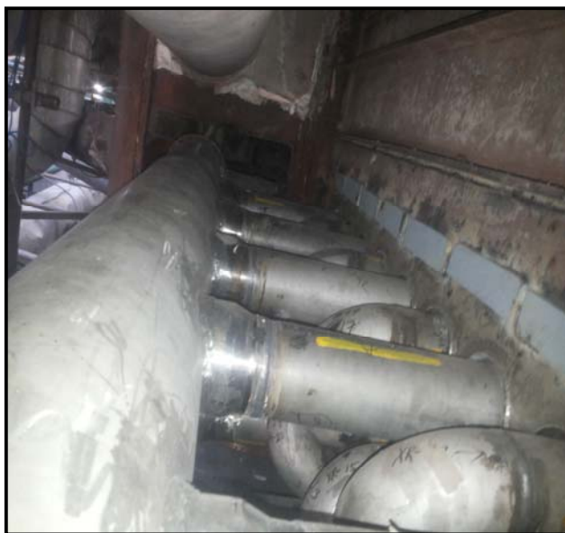
Header end of coil after header welding
