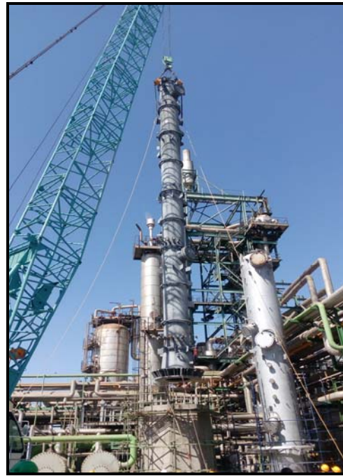
Erection of 1104-E
