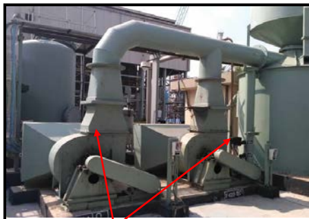
Old sliding gate valves
