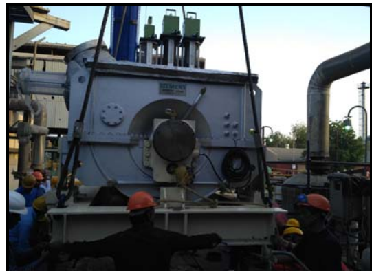
Turbine being positioned on foundation
