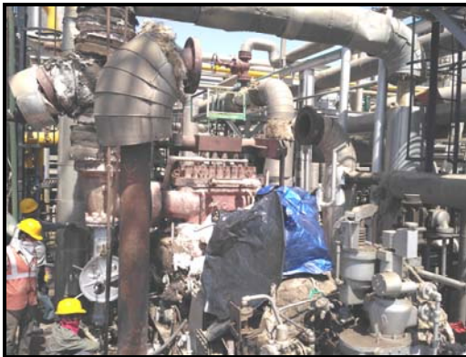
Removal of Steam Inlet & Extraction Piping
