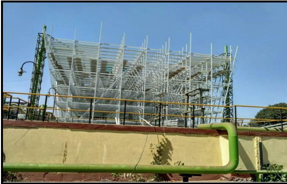
Erection of new FRP cooling tower structure - 2
