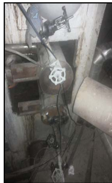
Header blinded for hydro test
