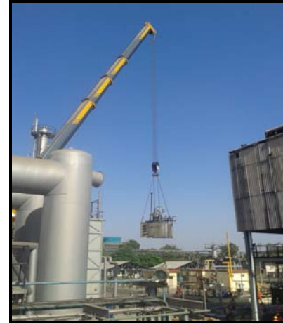
Dismantling & Removal of existing 101-J / 105-J LO console
