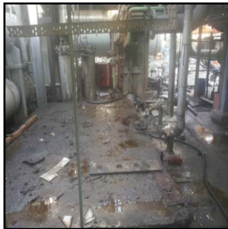
Foundation after removal of LO console
