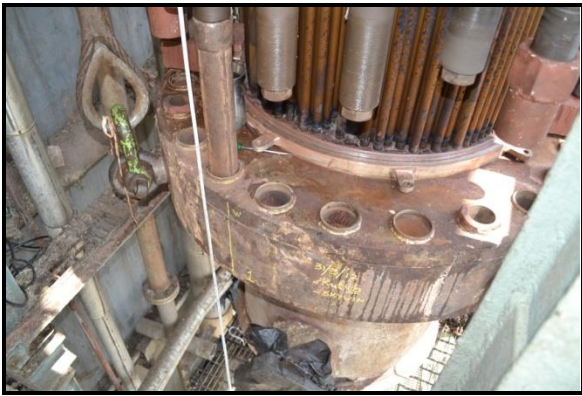
Tube bundle lowering after providing 4 nos. of guide
