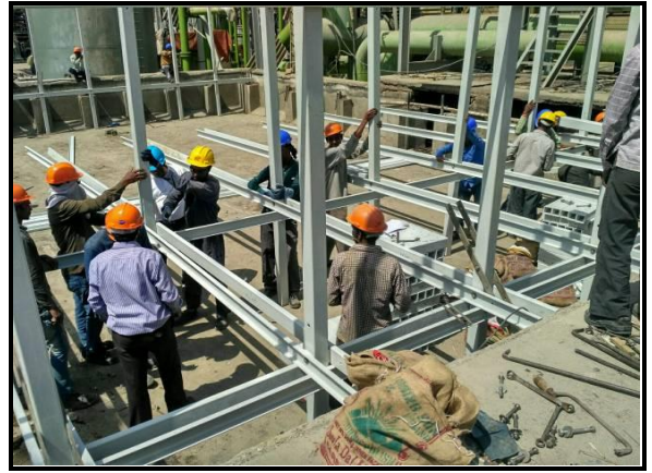
Erection of new FRP cooling tower structure - 1
