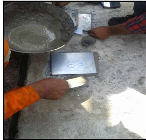
Fixing of Packer Plates using Shrinkomp
