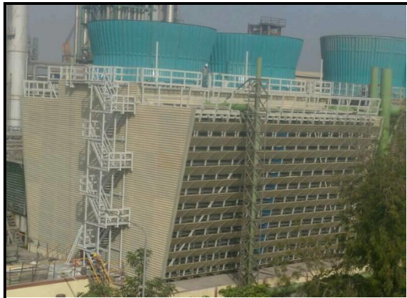
Completed New FRP Cooling Tower
