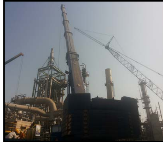
Erection of LO Console
