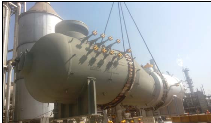
Erection of MP Boiler
