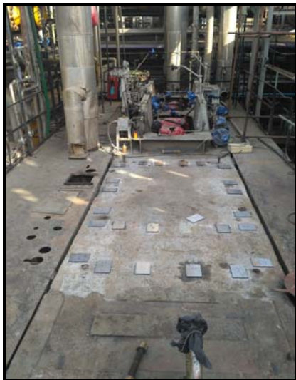
Surface Cleaned after Micro chipping & Blue checking
