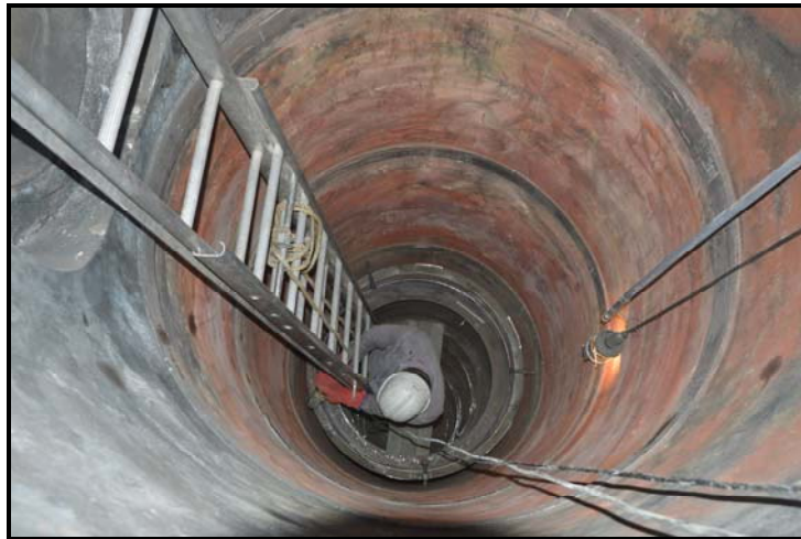
101-CA after complete removal of liner and refractory
