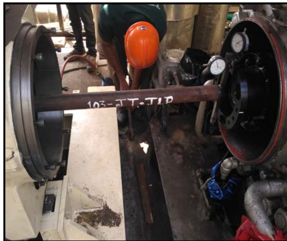
Alignment Fixture fixed
