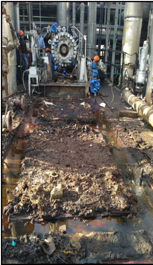
Turbine Floor Before cleaning
