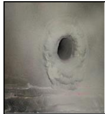
After final welding D.P.
