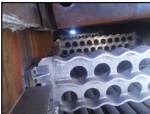
ITS placed in position
