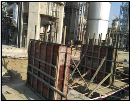
Template made for 1123-C
