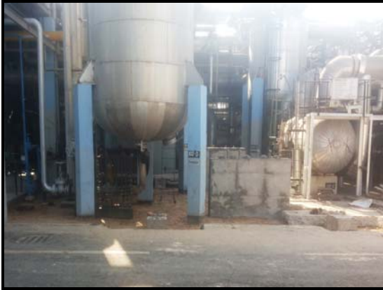
Foundation of 1114-CA/B ready and 1104-CA/B/C u/p
