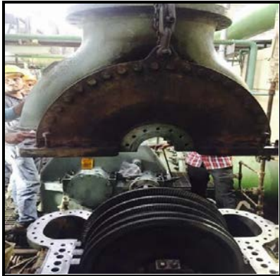
Top casing removal
