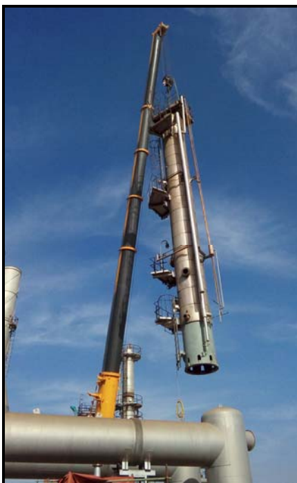
Removal of 104-E
