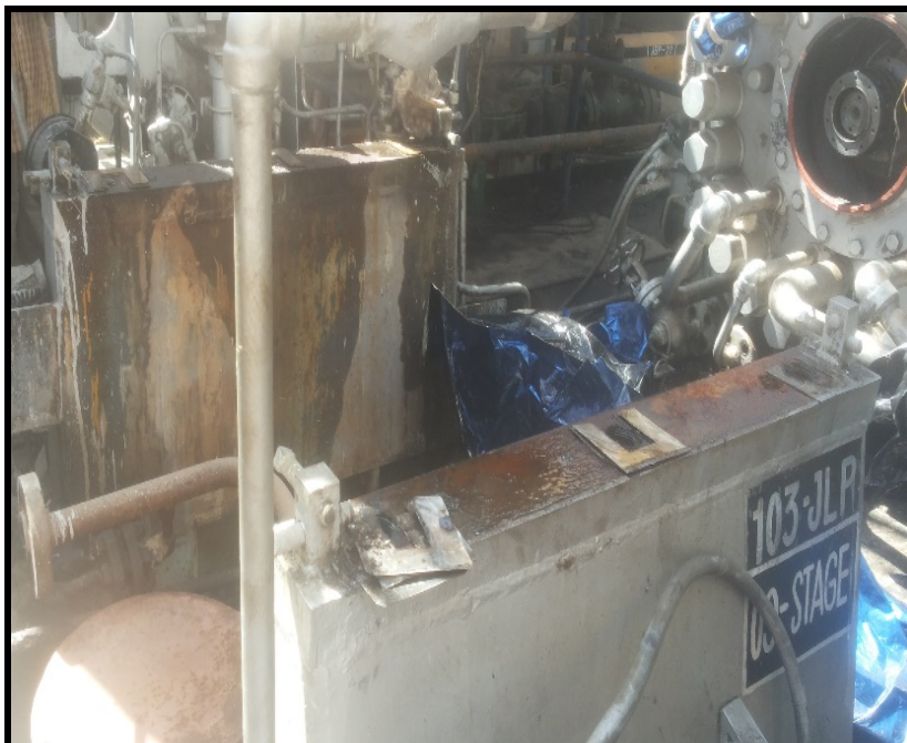
LP Compressor base after removal of compressor
