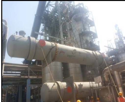
Erection of 1114-CA/B
