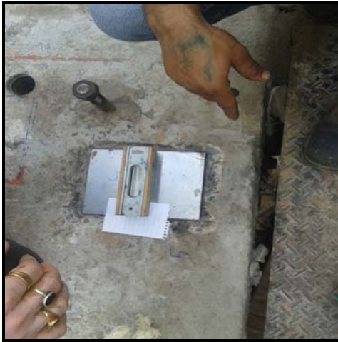
Packer Plate Level checking by Master Level
