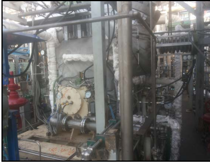
View of Turbine after completion of work
