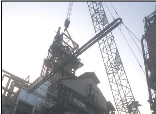
Coil lifted for installation
