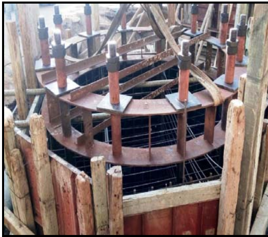
Template of 114-D in position
