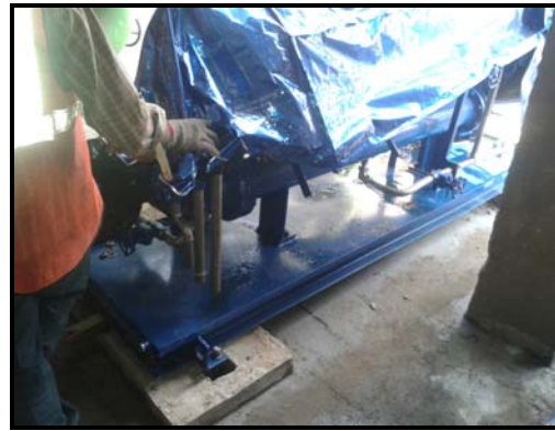
Erection of HP Oil Cooler
