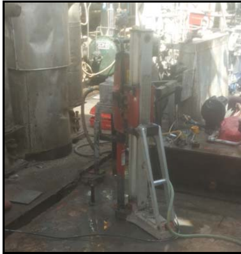
Core cutting for M 36 bolts
