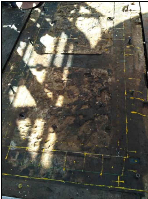
Packer Plate positions marked on floor
