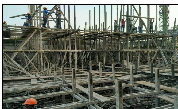
Dismantling of old wooden cooling tower structure-3
