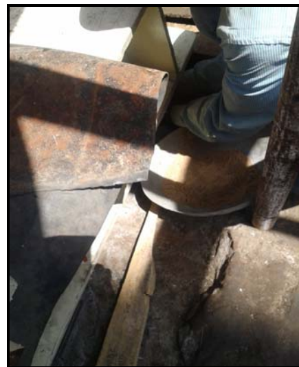
Sand filling in the pockets of foundation holes
