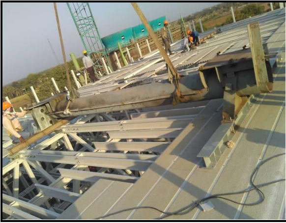
Erection of SS torque tube
