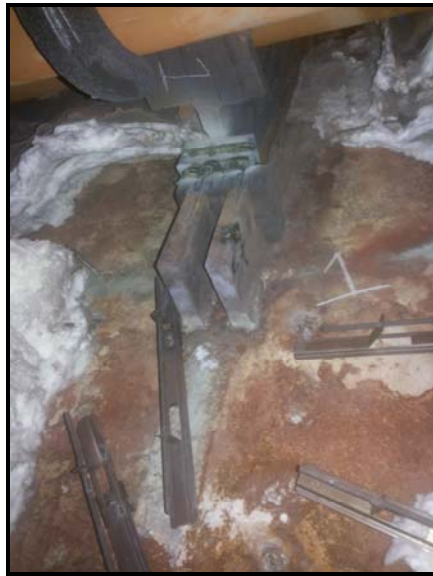
1st ITS support after repair
