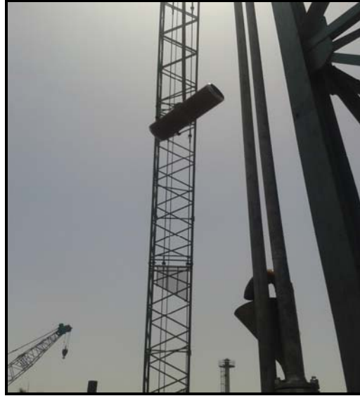
Flow nozzle of Extraction Line lifted
