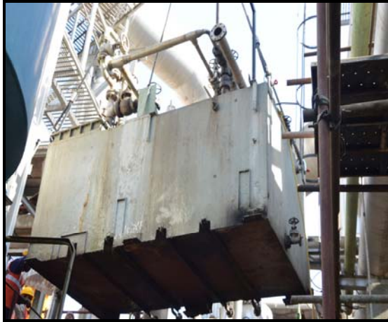
Dismantling & Removal of existing 101-J / 105-J LO console
