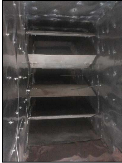
PRC-23 dampener area after replacement of dampener and CF insulation
