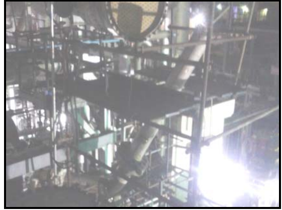
Blowing arrangement of Steam inlet line
