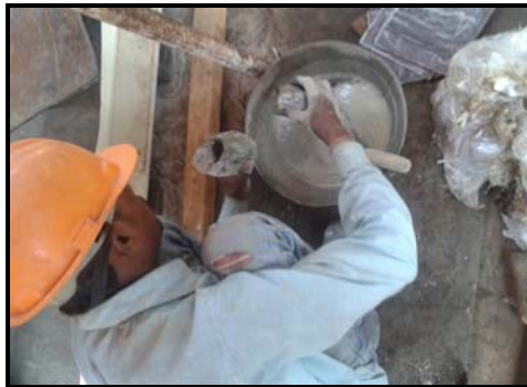
Shrinkkomp filling in the pockets of foundation holes
