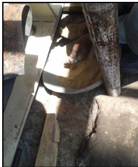
Sand filling in the pockets of foundation holes
