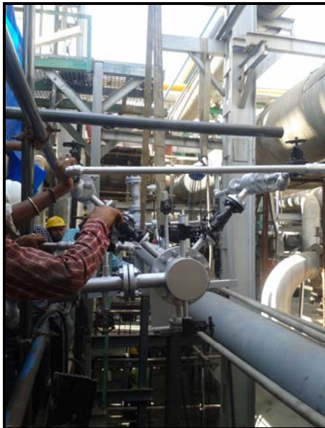
Gland Steam Condenser erected on 26/03/2017
