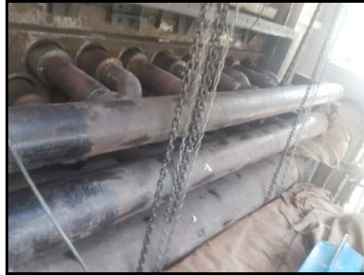
Outlet header after final welding
