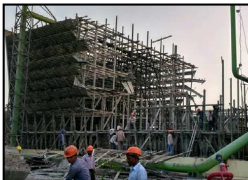
Dismantling of old wooden cooling tower structure-2
