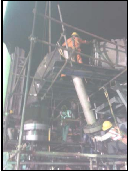
Blowing arrangement of Steam inlet line
