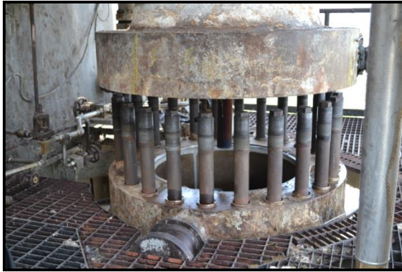
Lifting of top dome – up to stud
