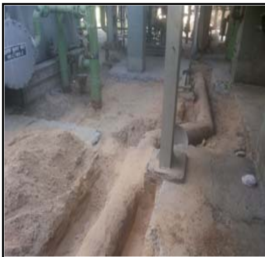
Excavation job for foundation and CW lines modification
