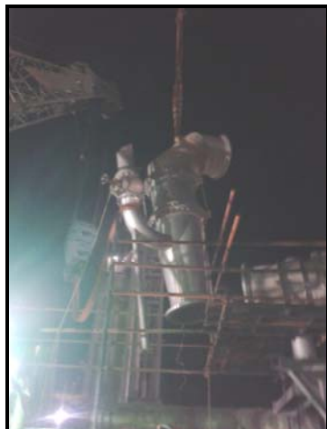
Removal of Exhaust Piping
