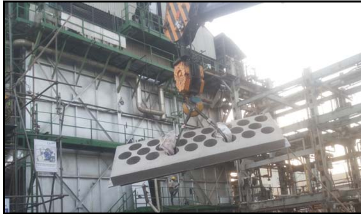
Erection of End tube sheet
