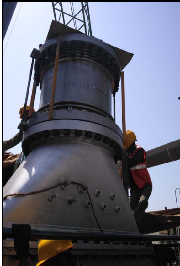
Installation of Expansion Bellow
