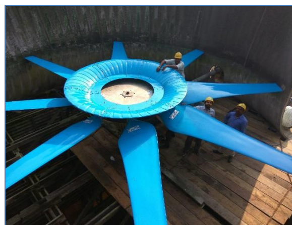
New Fan blade assembly with seal disk
