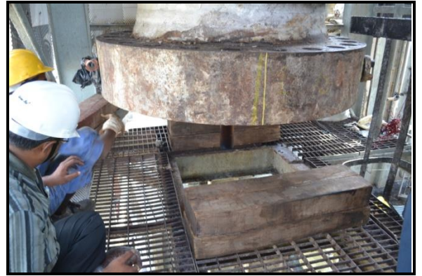
Placing of top dome
