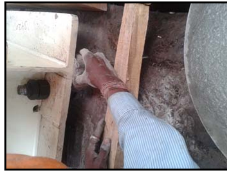
Shrinkkomp filling in the pockets of foundation holes
