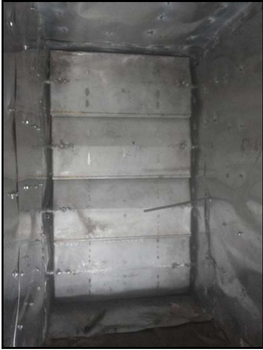
PRC-23 dampener area after replacement of dampener and CF insulation
