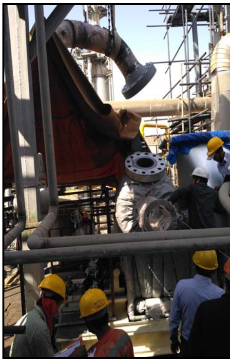
Inlet Line Fabrication u/p
