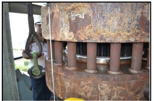
Lowering of tube bundle
