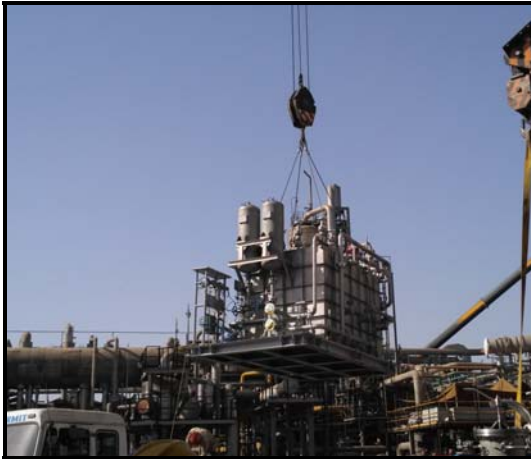
Lifting of new 101-J/105-J LO Console for Erection
