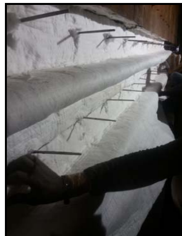
Insulation provided on wall
