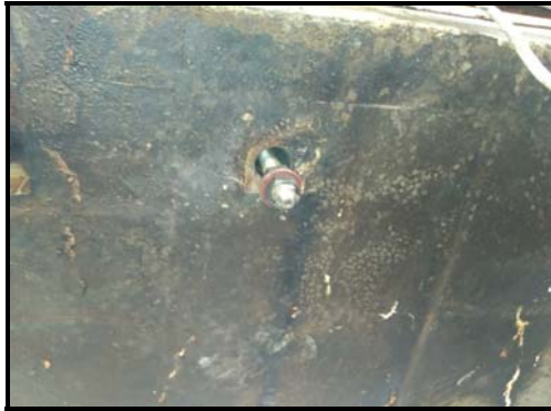
Foundation bolt exposed from bottom
