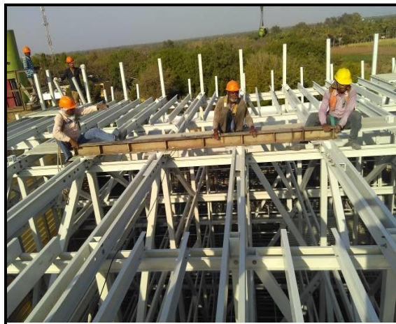
Erection of SS I-beam ( gear box side )
