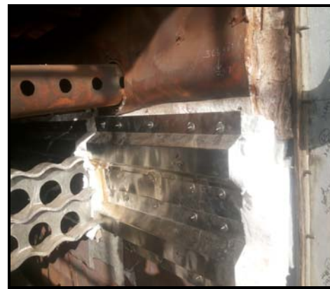
Corbel provided on wall # 5
