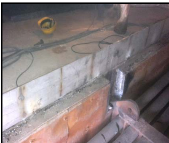
Provision for installation of ITS support and guides on wall 6
