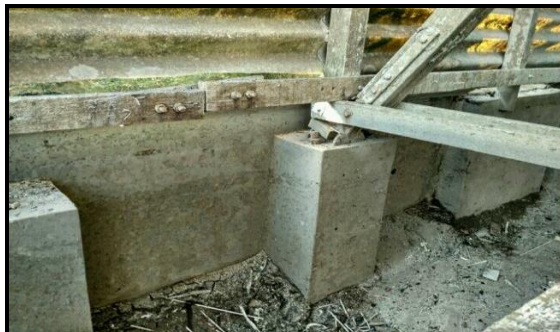
Base casting with RCC pedestal in basin
