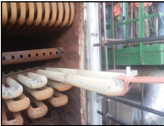
Removal of Coil under progress
