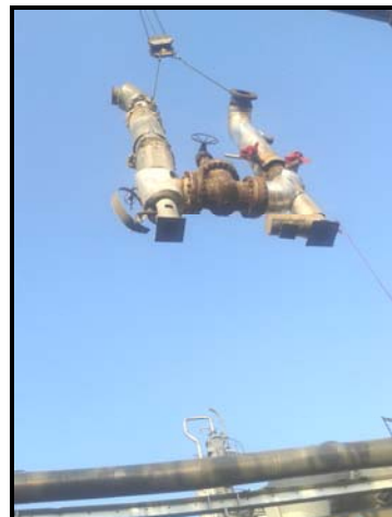
Removal of Extraction I/V
