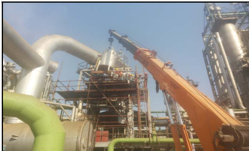
Erection of 101-J RD Tank
