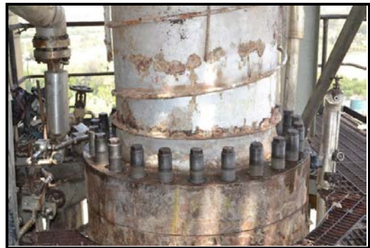
Top dome flange – after nut removal
