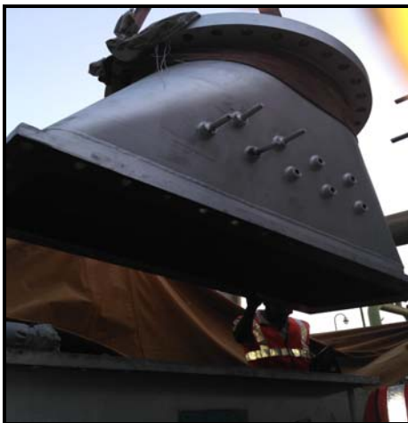
Installation of Transition Piece
