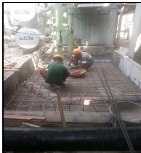
Foundation job of pump and drives under progress
