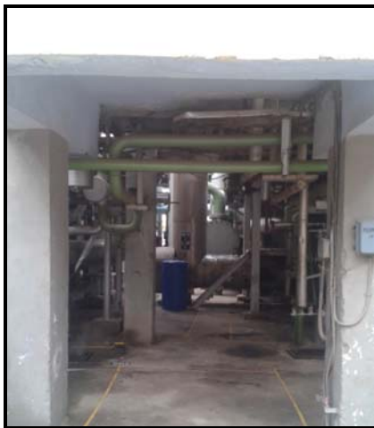
Marking of Foundation Layout of HP Oil system and Accumulator
