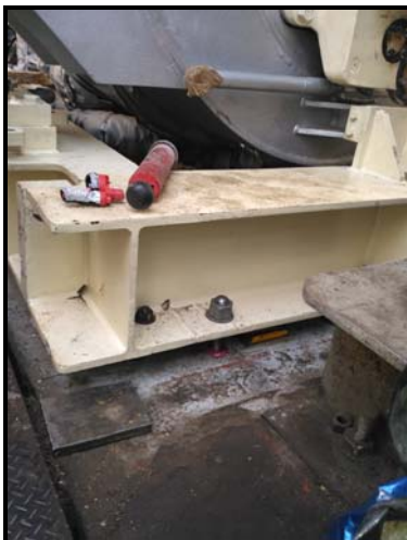
Grouting of front 2 bolts using Hilti Chemical
