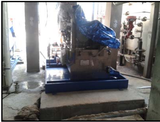
Erection of HP Control Oil Console
