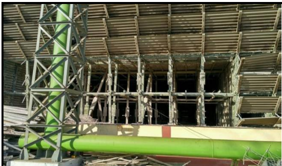
Dismantling of old wooden cooling tower structure-1
