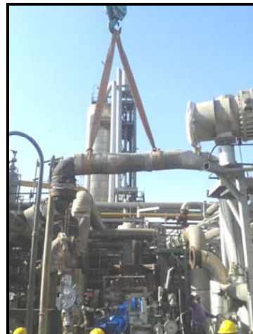
Removal of Steam Inlet & Extraction Piping
