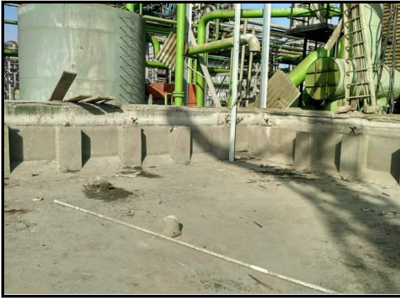
Complete dismantling of old wooden cooling tower structure
