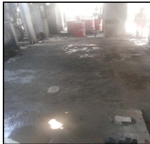
Foundation of LO console after breaking of top portion
