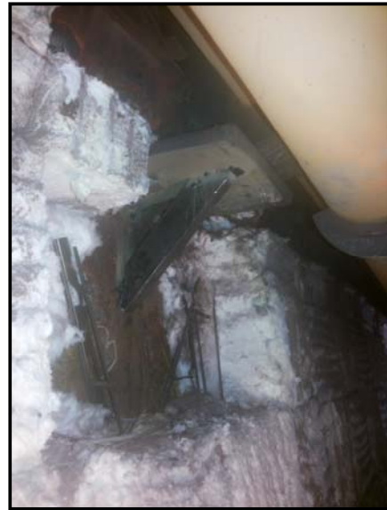
3rd ITS support after repair
