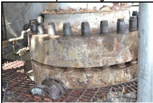
Lifting of top dome
