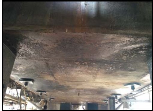
Lock Plate fixed from bottom
