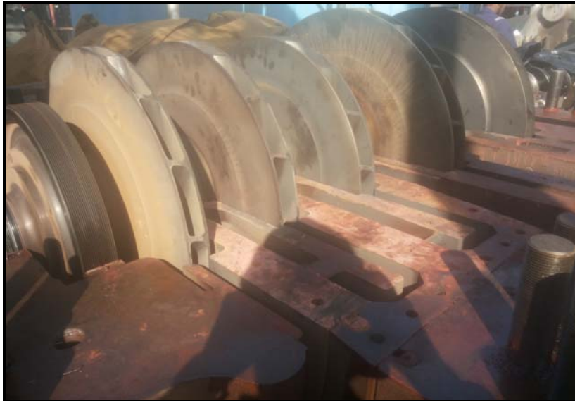
Rotor after removal of top casing
