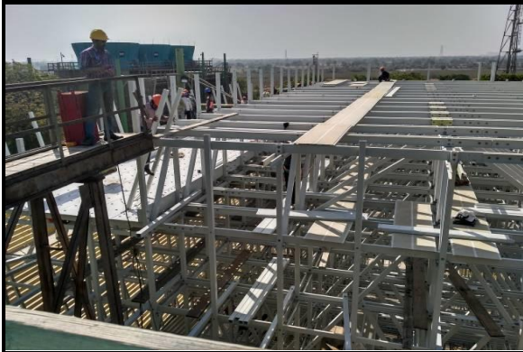
Erection of hot water distribution deck
