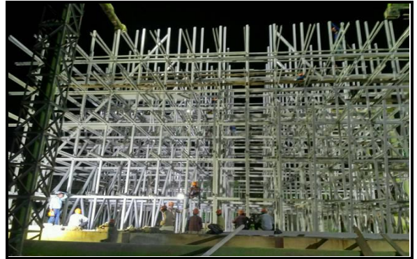
Erection of new FRP cooling tower structure - 3
