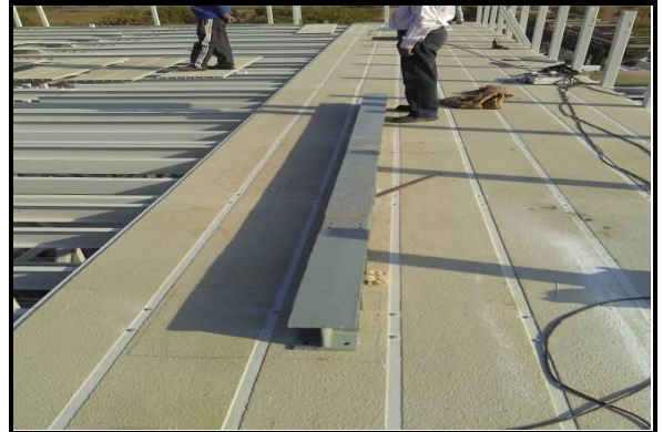
Erection of fen deck
