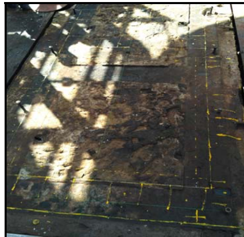
Marking of New Turbine Base frame layout on floor
