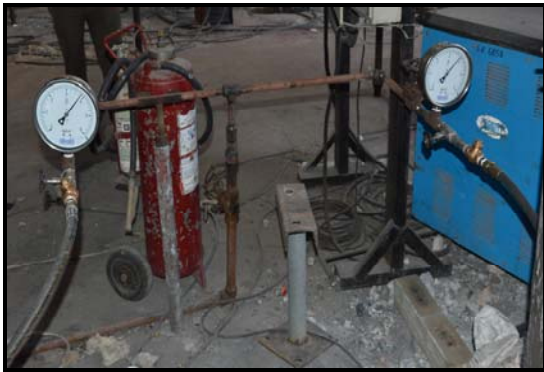
NG line taken from GAIL and connected to 101 CA & B
