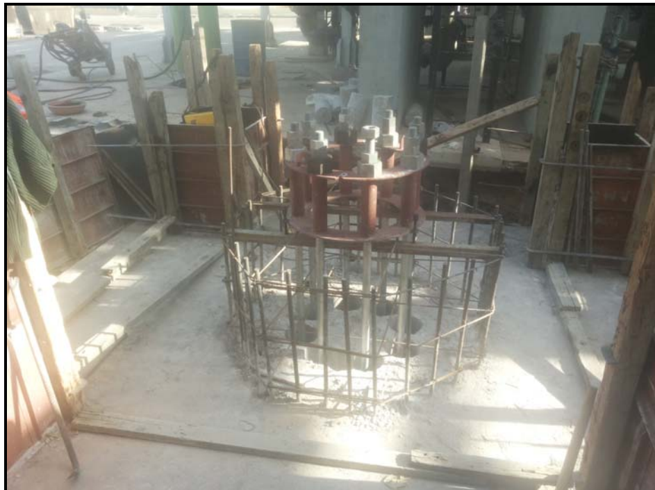
Template of 106-E provided in foundation
