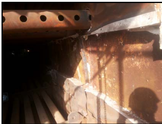
Insulation removed on wall #5
