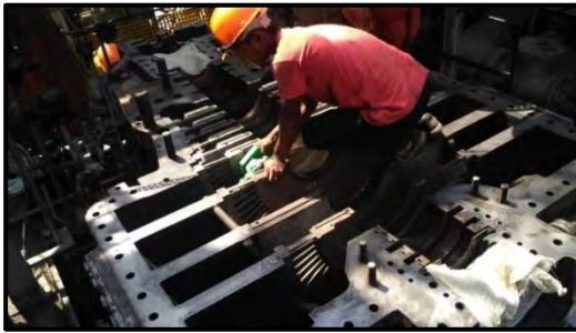
Final Cleaning of bottom casing half before Assly.
