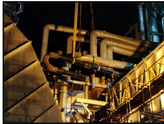
Lifting of outlet spool piece with elbow
