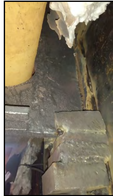
Supports after repair
