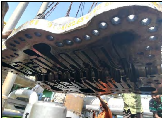
105-JHP Top Casing Half Removal
