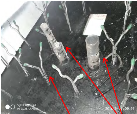
Bitiminius painting, new anchor & old piping (for draft measurement)
