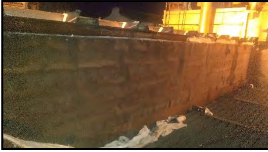
South side wall above LT coil
