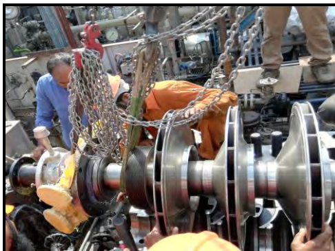
Setting of Mech. Seal during placement of Rotor
