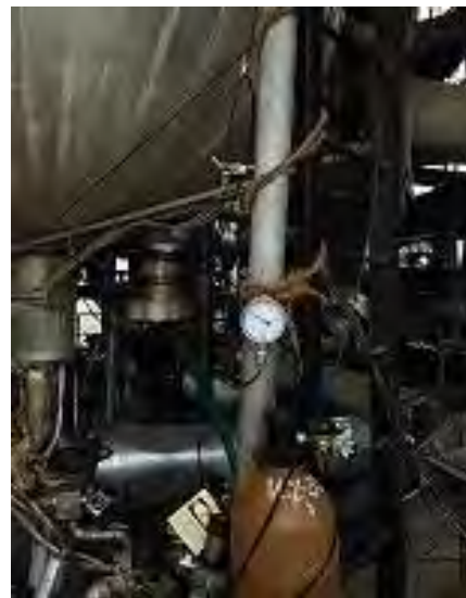
WATER SEAL ARRANGMENT SET AT 0.3Kg/cm 2
