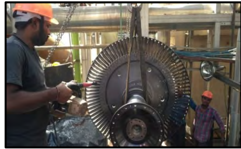
Final Cleaning of Rotor before Assembly
