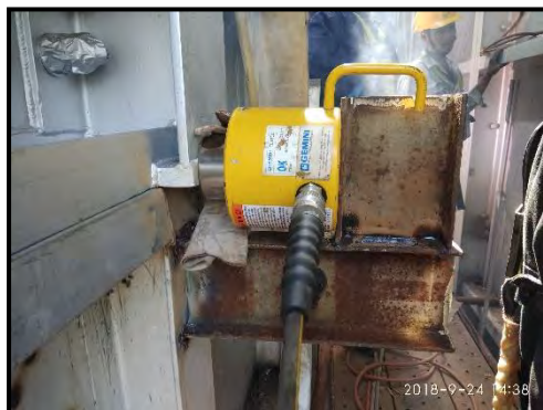
North side channel levelling before welding
