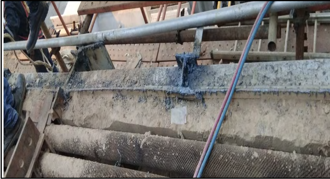
South side channel after cutting
