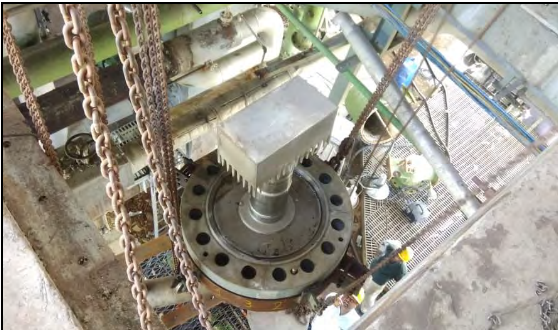
BOTTOM COVER REMOVED & PLACED ON 2 nd FLOOR
