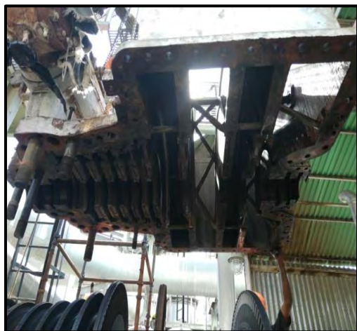
Removal of 101-JT Top Casing Half
