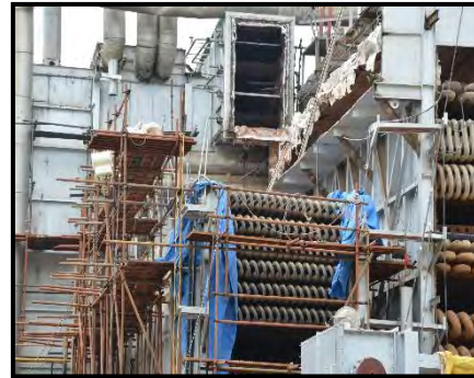
After removal of side walls @ 6804
