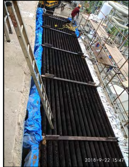
After hydro jetting
