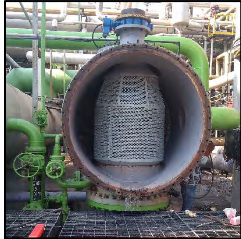
Strainer assembled after cleaning
