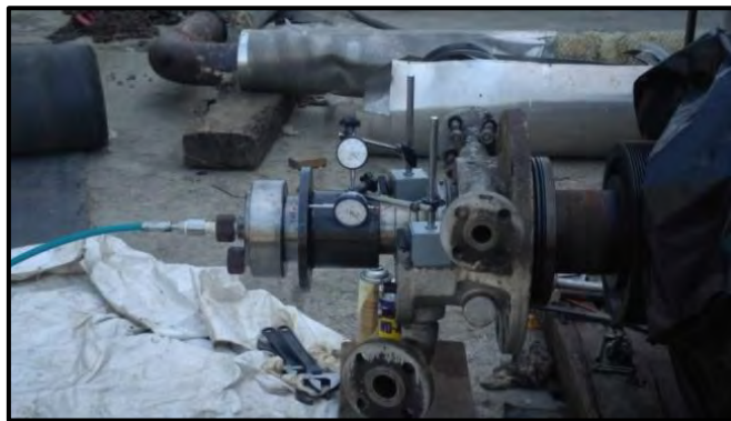
Coupling Hub Removal from shaft
