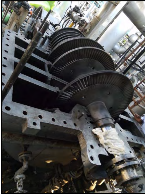
Rotor placed on bottom casing half
