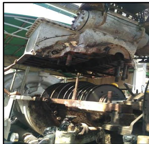
Removal of 101-JT Top Casing Half
