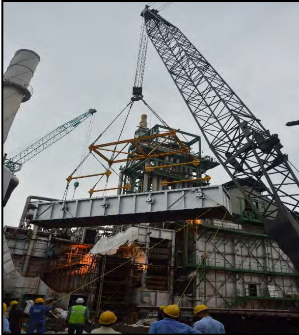
New LT coil module Erecting
