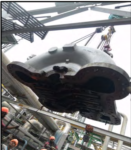
Lifting of 105-JLP Top Casing half
