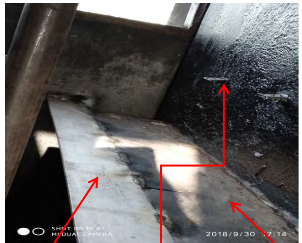
New SS304 plate welded with old retainer plate & hooks for brick holder pin
