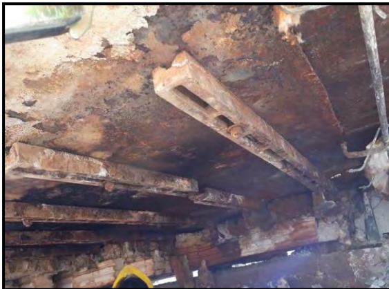
Top roof Hanging bricks after removal
