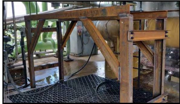
FABRICATED FRAME FOR BOTTOM COVER
