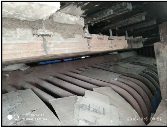
Roof Brick installation under progress
