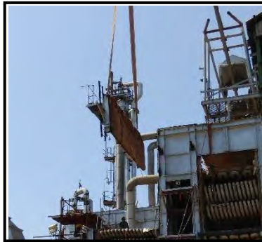
Side wall removal
