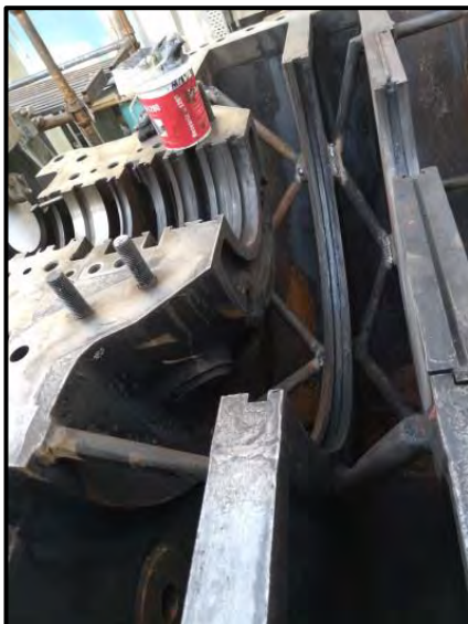
Weld Repaired Eroded Reinforcement Rods
