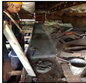
Filling of refractory over the bridge plate
