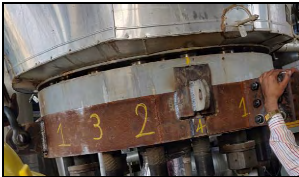
CLAMP FOR BOTTOM CHANNEL FLANGE & SAFFOLDING FOR BOTTOM SCAFFOLDING
