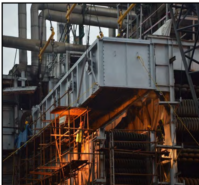
While placing in position
