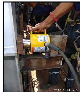
North side channel levelling before welding
