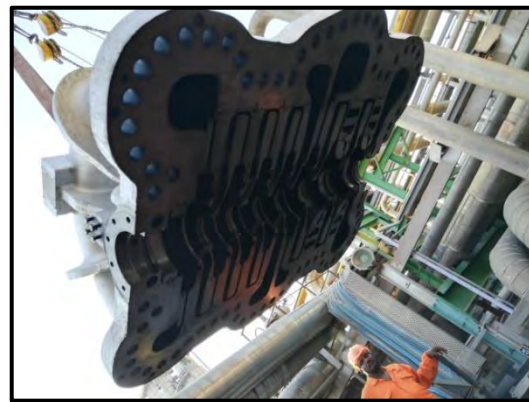
Placement of Top casing half for final Assy.
