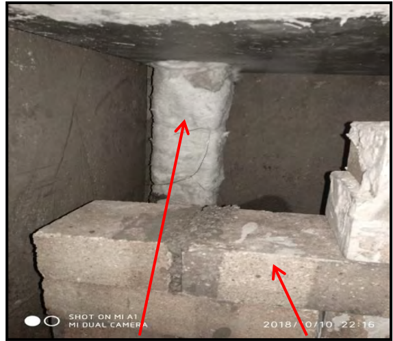
Ceramic fibre blanket and tunnel dense brick
