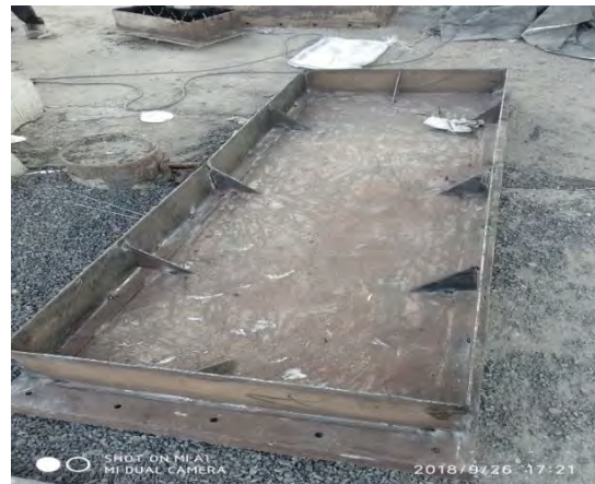
Welding of side plate and retainer with old removed panel
