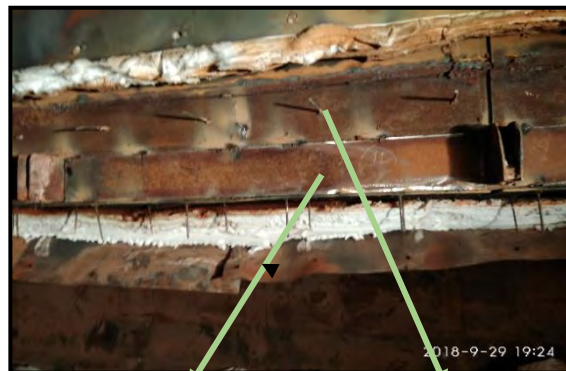
Welding with 6 mm plate & inconel studs
