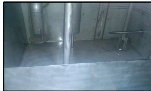
101-BJT LO console after cleaning
