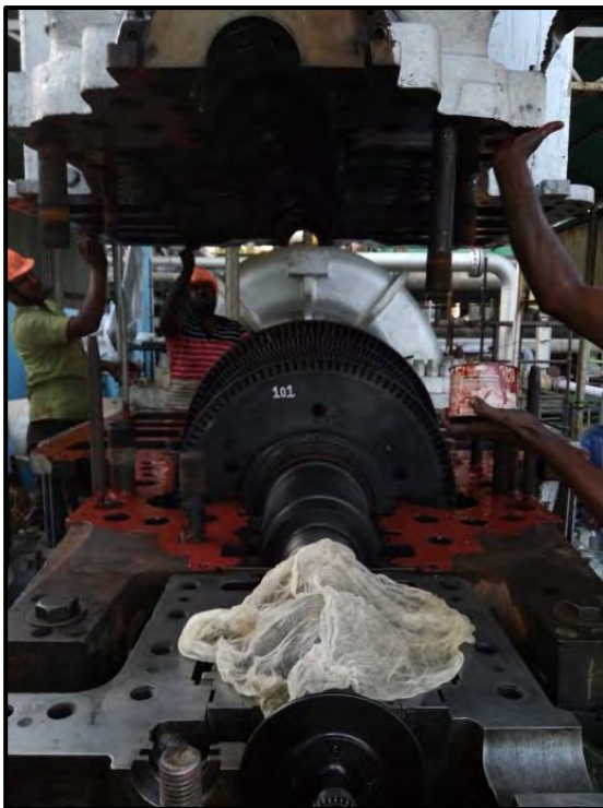
Application of sealing compound on parting plane
