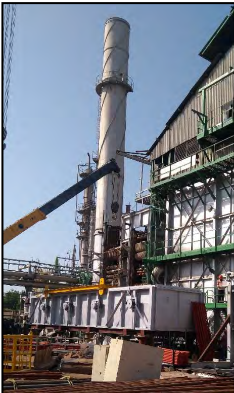
LT Coil was unloaded near Reformer/ Convection section
