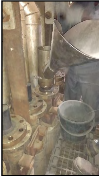
Catalyst loading by Dense loading method
