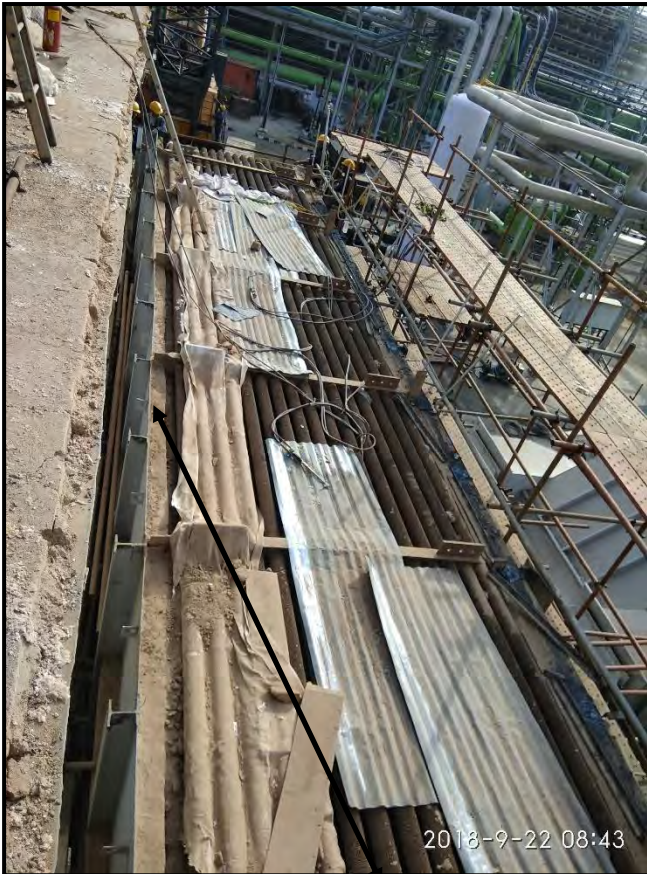
North side wall before channel welding
