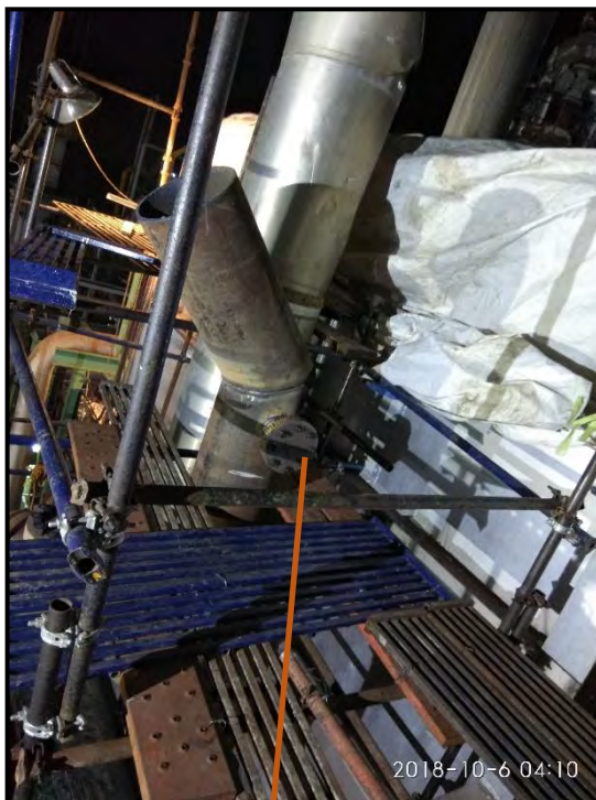
16" elbow welded to inlet header of coil for Blow stack
