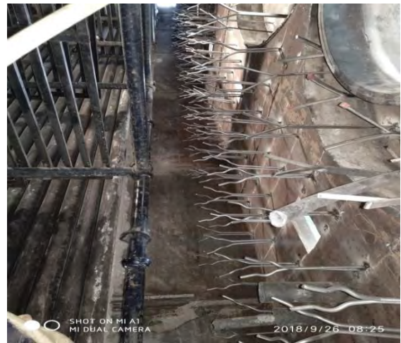
Anchor welding in burner block area
