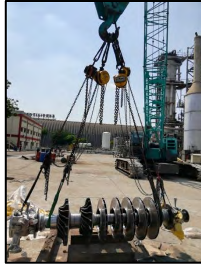
Lifting of Rotor for Assy. into casing
