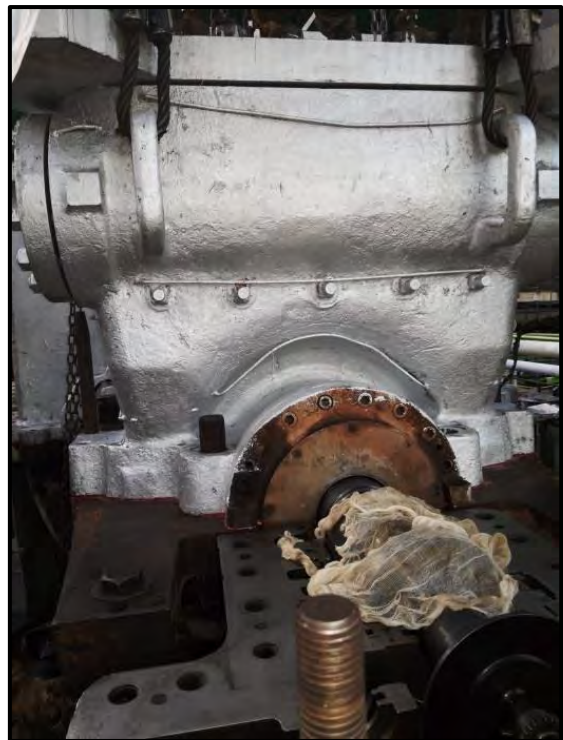
Placement of top casing on bottom casing
