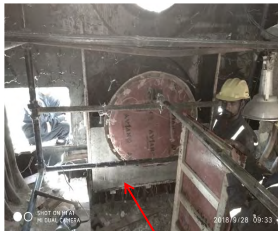
Castable lining of bottom half of 1 st burner (bottom most)
