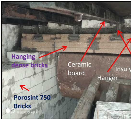
Top roof with Burner wall
