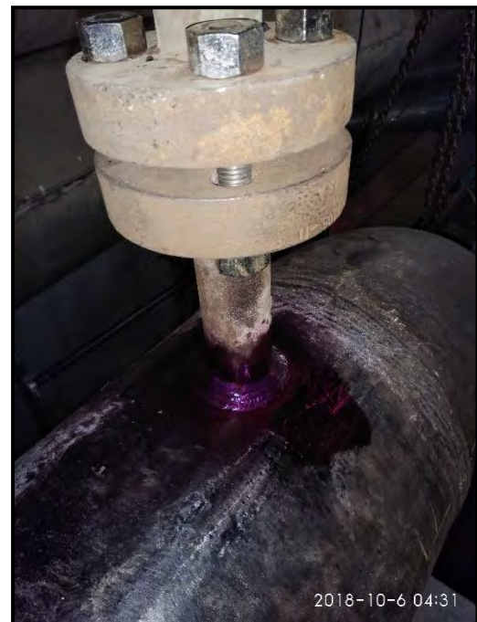
DP after welding
