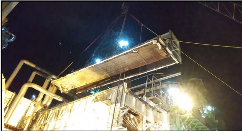
Lifting of LT panel with transition zone
