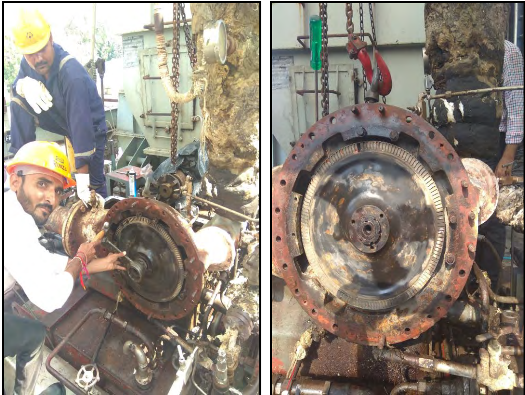
FD Fan Turbine during overhauling
