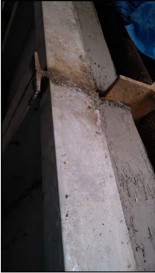
New Refractory on side wall of BFW coil
