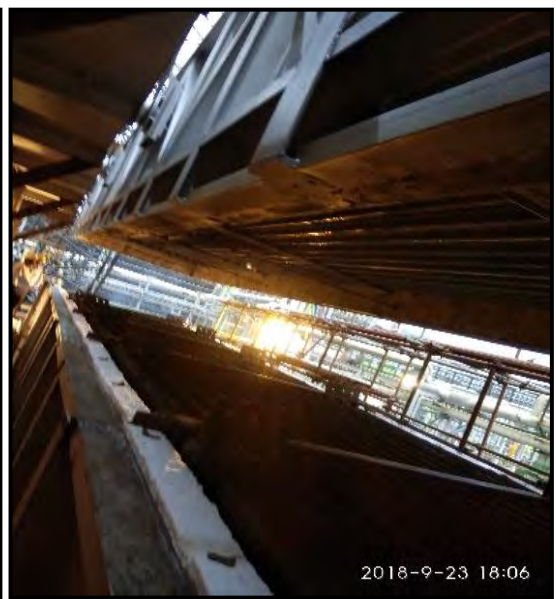
Refractory placed b/w the modules
