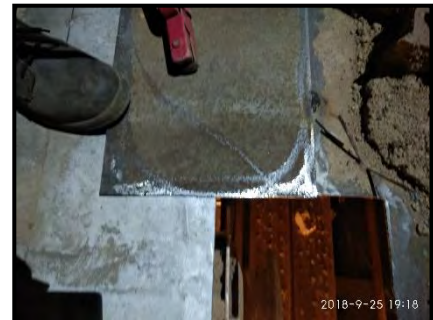
Bridge plate welding
