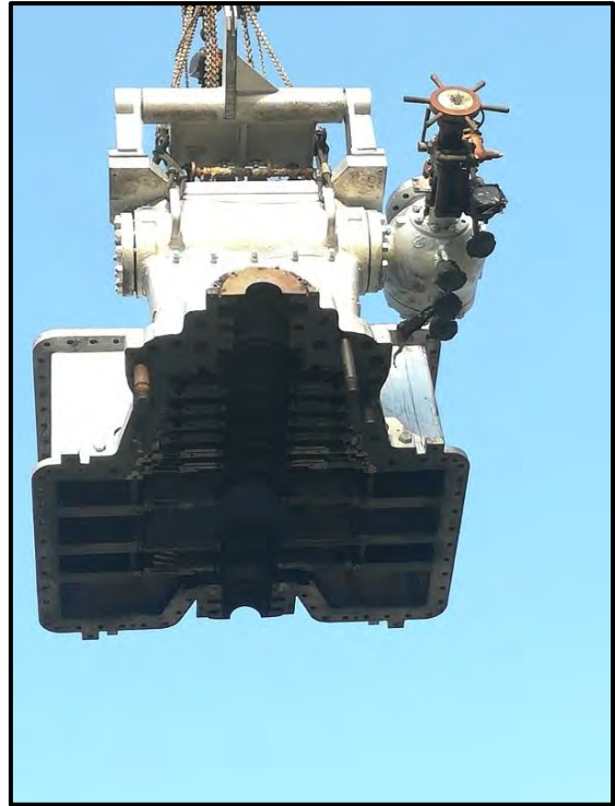
Lifted Top casing half for Assy.
