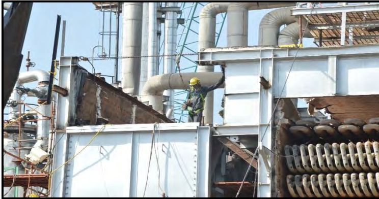
South Side wall above new Lt coil module
