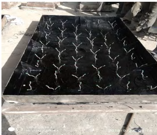
Panel after welding of Anchors and bituminous painting
