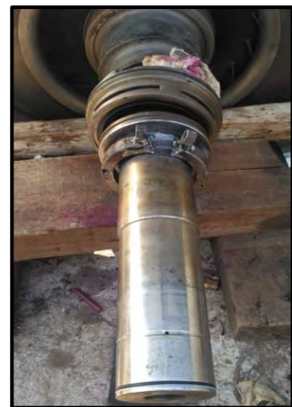
Lock nut cut for Seal Collar removal as it was stuck
