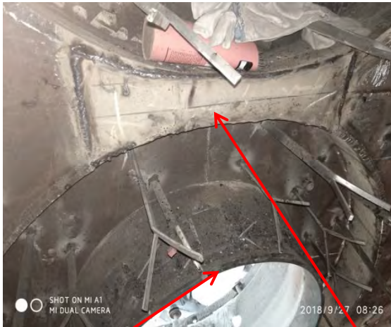
New anchor welded in burner block area & Patch plate
