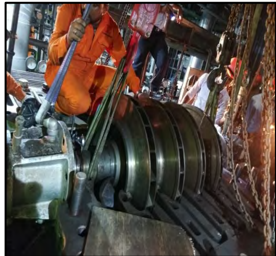
Lifting of 105-JLP Rotor
