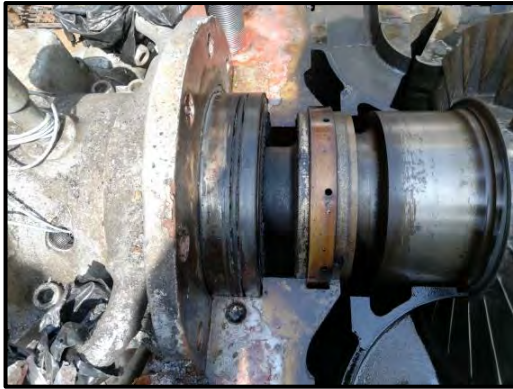
Bearing Housing and Mech. Seal Assy. at NDE
