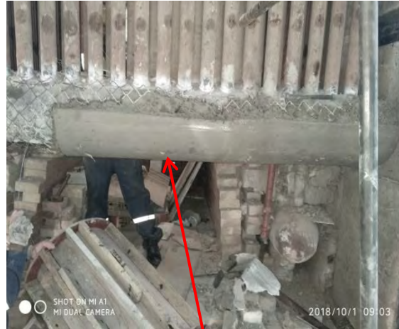
Castable lining of Coil C header (Under progress)
