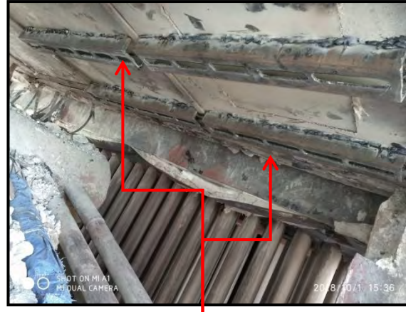
New channel welded with top roof
