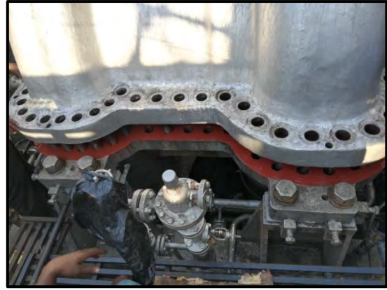
Top casing Half placement at bottom casing half
