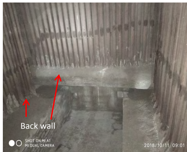
Partition wall & bridge walls
