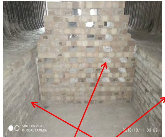
Partition wall & bridge walls
