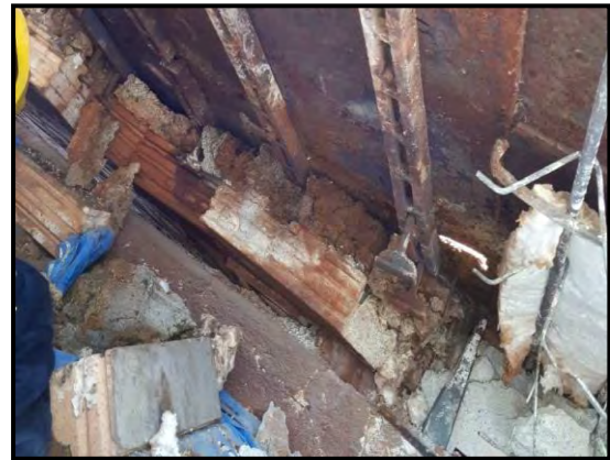
Top roof Hanging bricks after removal
