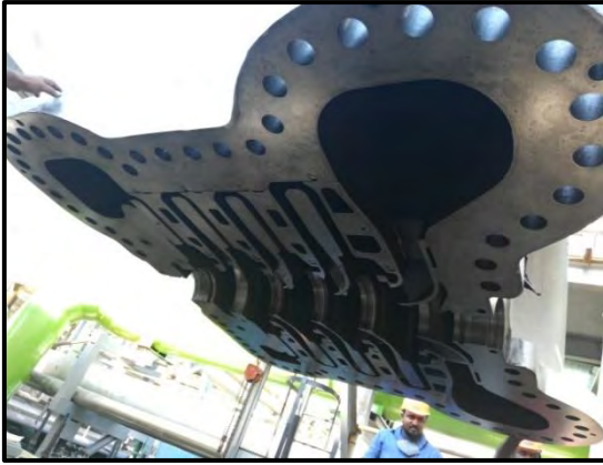
Top casing Half placement at bottom casing half
