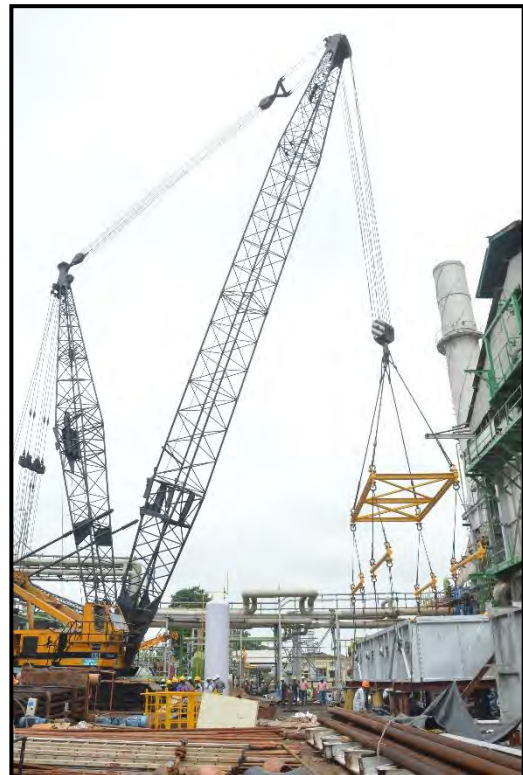
LT Coil was unloaded near Reformer/ Convection section
