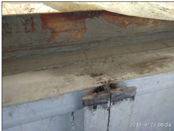
North side refractory
