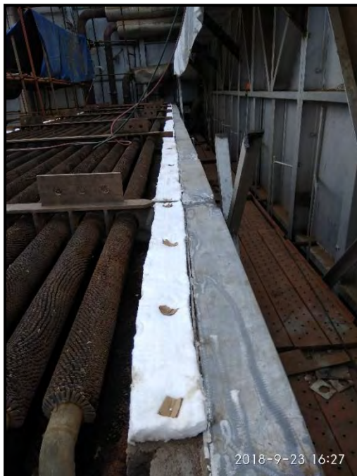
Blankets placed towards north side wall
