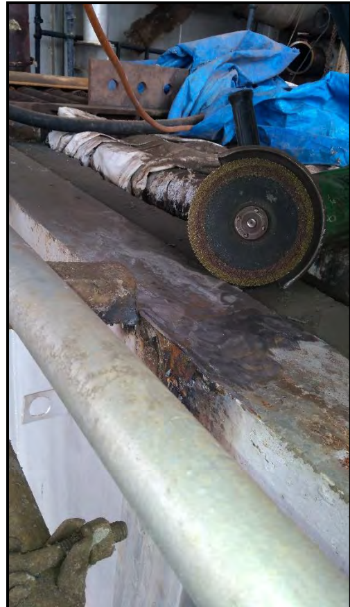
Grinding of south side channel
