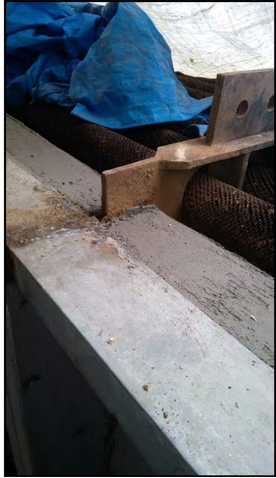
New Refractory on side wall of BFW coil
