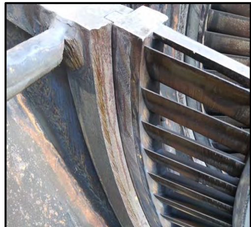
Eroded Reinforcement Rod
