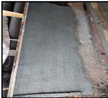
Filling of refractory over the bridge plate
