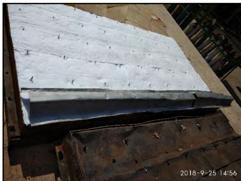
new blanket and panel cover
