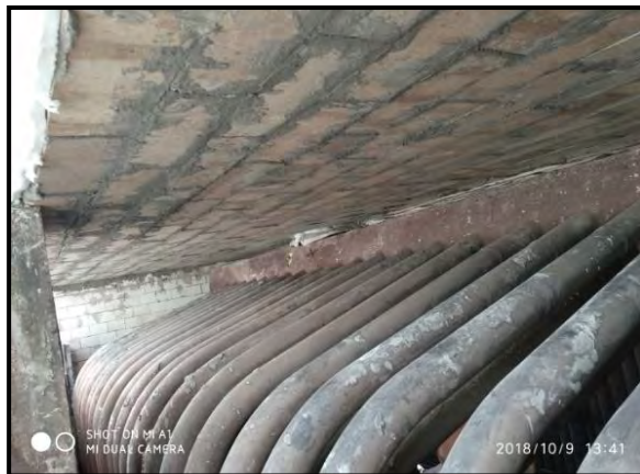
Top roof bricks
