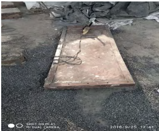
Panel after cutting of side plates
