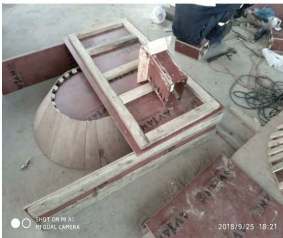
Wooden formwork preparation for castable burner block
