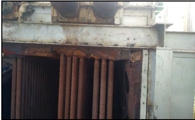
View of Coil C,D & E after removal of Wall #10
