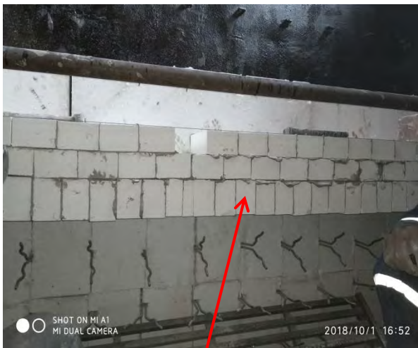
Porosint 750 bricks ( bottom most )
