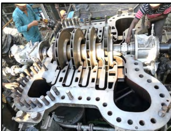
Clearance Measurement after Rotor placement & prepared for casing assembly
