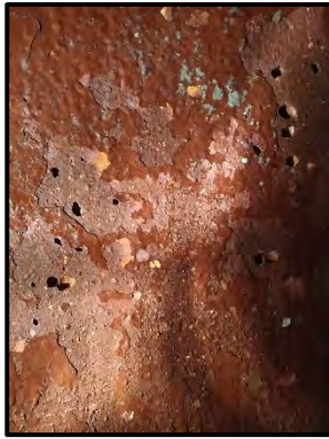
Cavities observed in Epoxy at scattered locations
