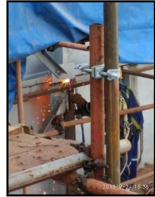
Welding of side wall
