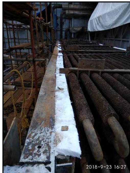
Blankets placed towards south side
