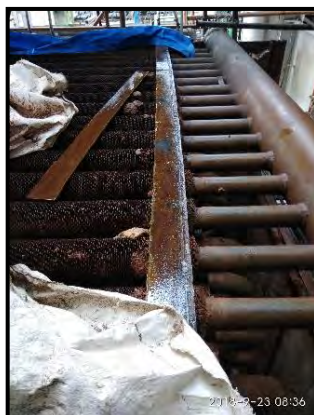
After strip welding
