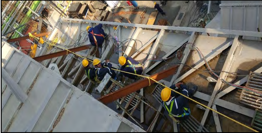
Beams were welded between LT section Roof and transition zone.
