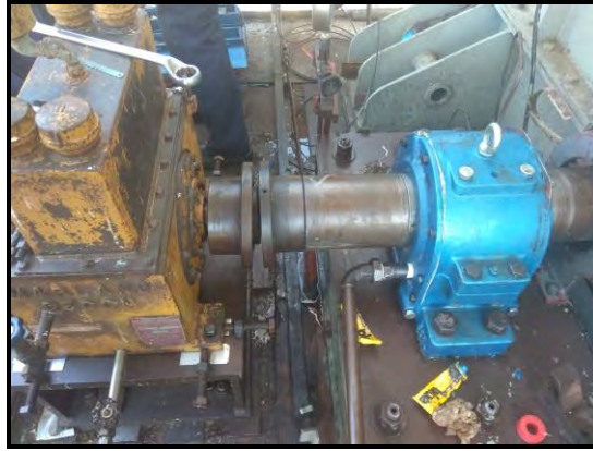
New Plumber Block
