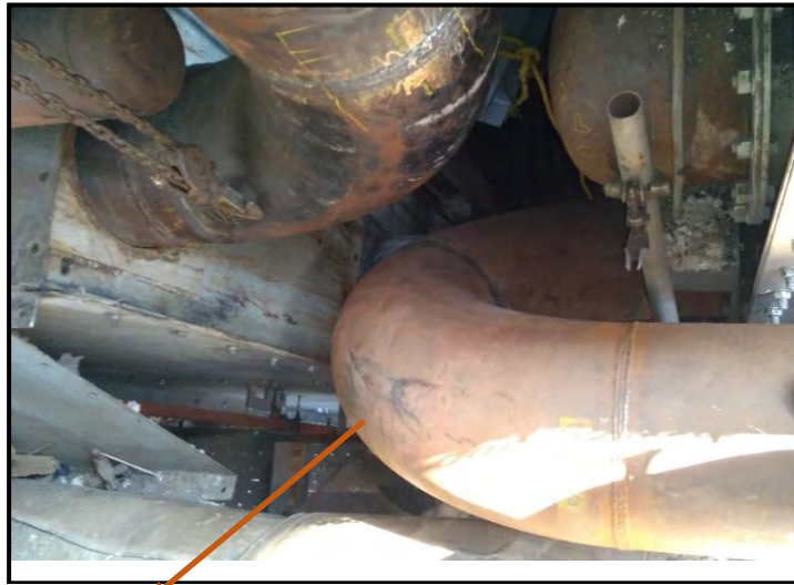
16" elbow welded to inlet header of coil for Blow stack
