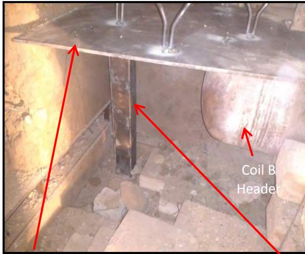
Retainer plate for tunnel brick & castable and support
